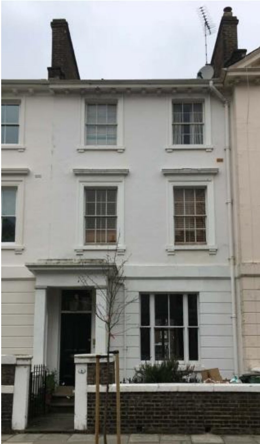
1. Front elevation of No. 1 St Mark's Crescent
