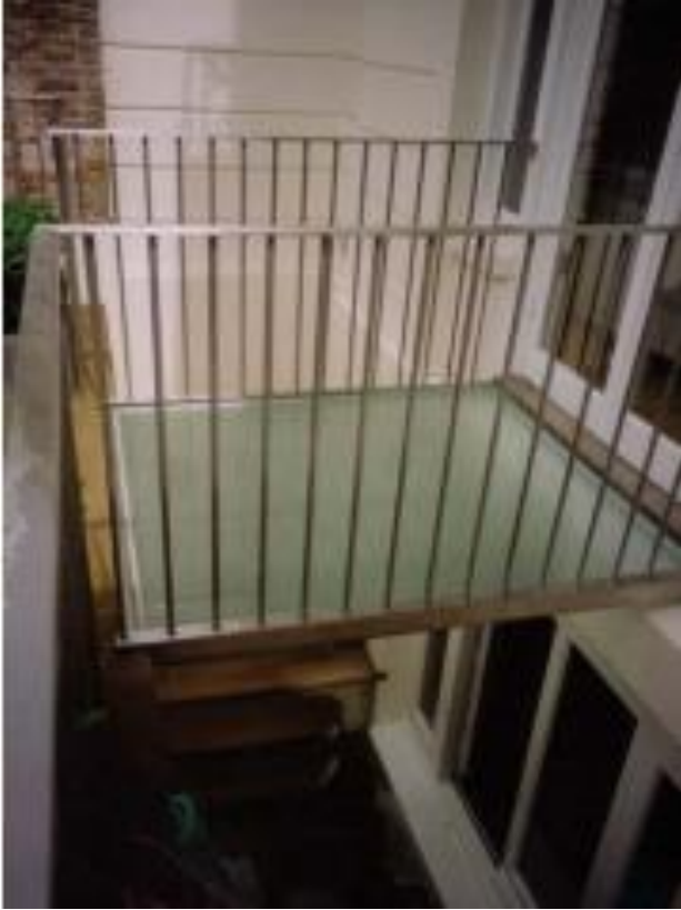
6. Example of glazed bridge
