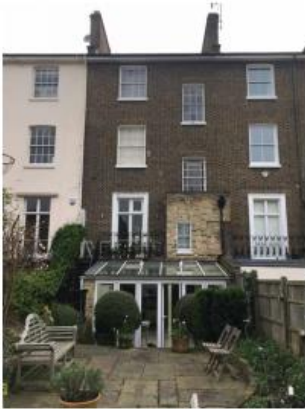
2. Rear elevation of No. 1 St Mark's Crescent
