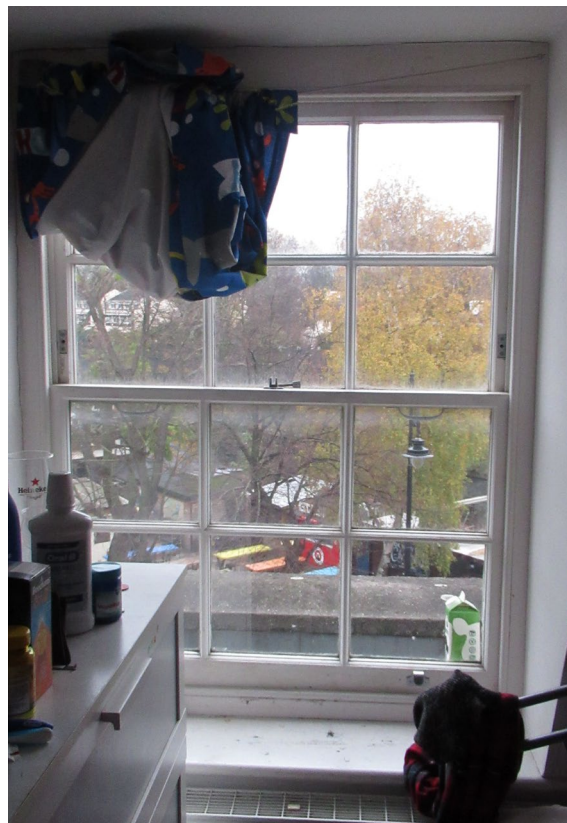
Figure 14: Internal view of window at third floor level – Bedroom D
