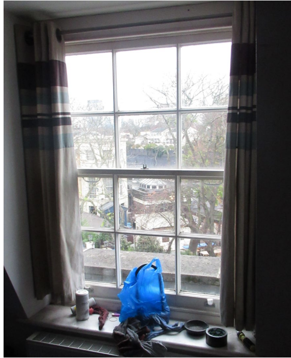
Figure 13: Internal view of window at third floor level – Bedroom C
