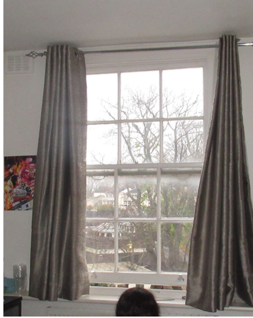
Figure 11: Internal view of window at second floor level – Bedroom A
