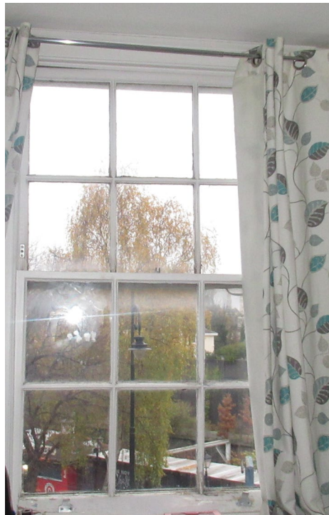
Figure 12: Internal view of window at second floor level – Bedroom B
