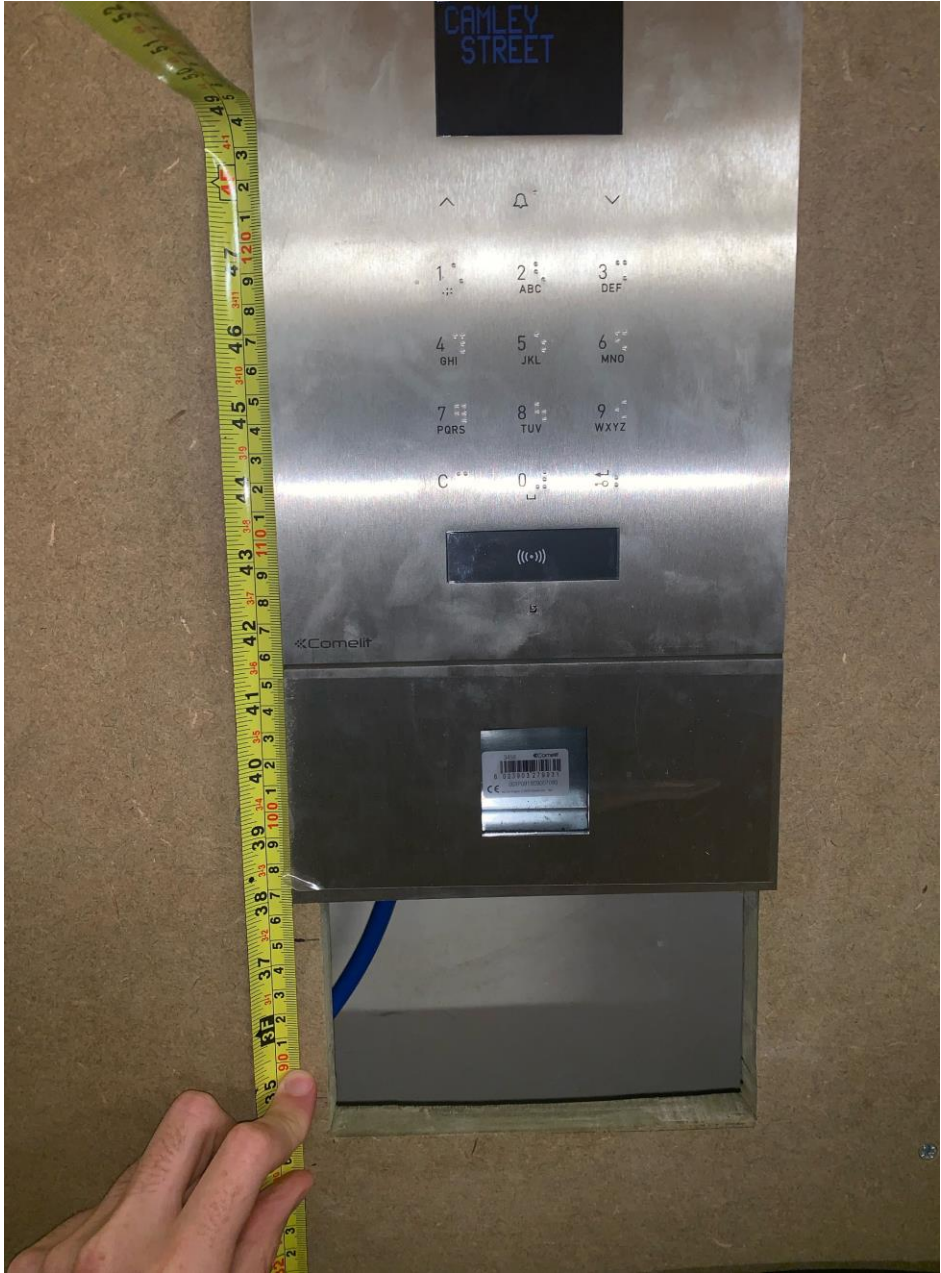
keypad controls are between 1000mm – 1200mm AFFL
