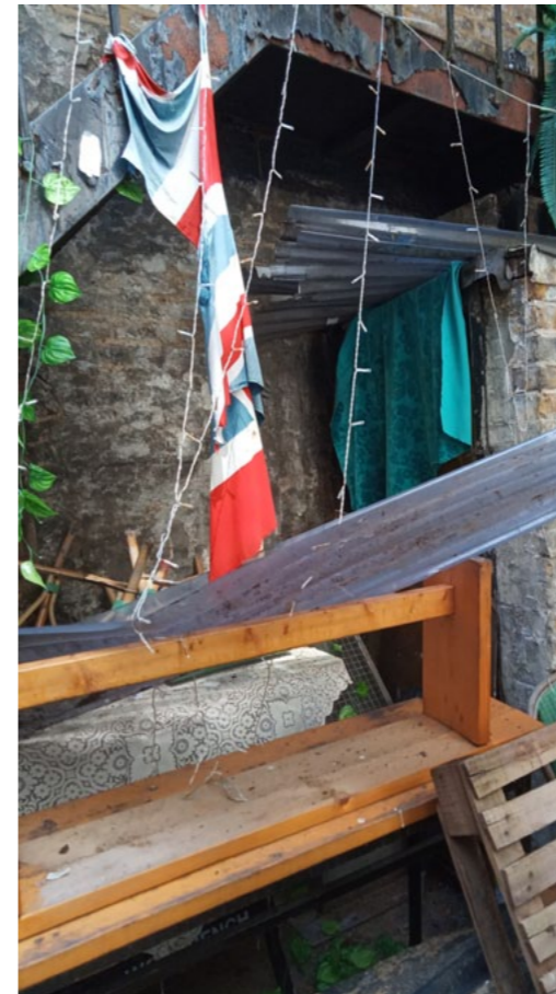
Fig 10. Ext.. Store to be refurbished
