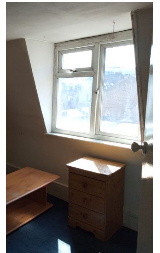
Fig 25. Existing rear window to be replaced in existing opening
