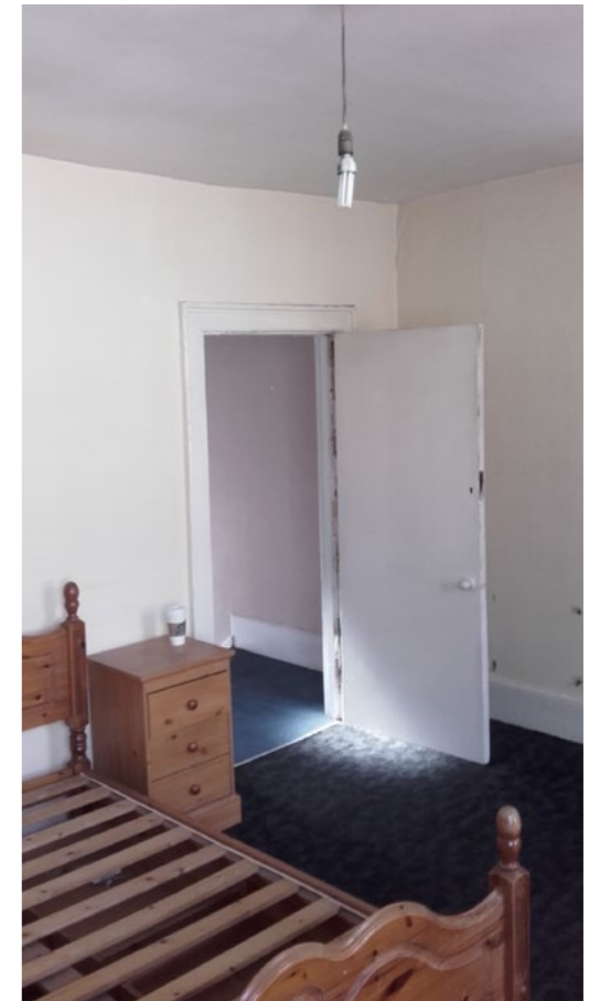
Fig 19. All flush doors replaced
