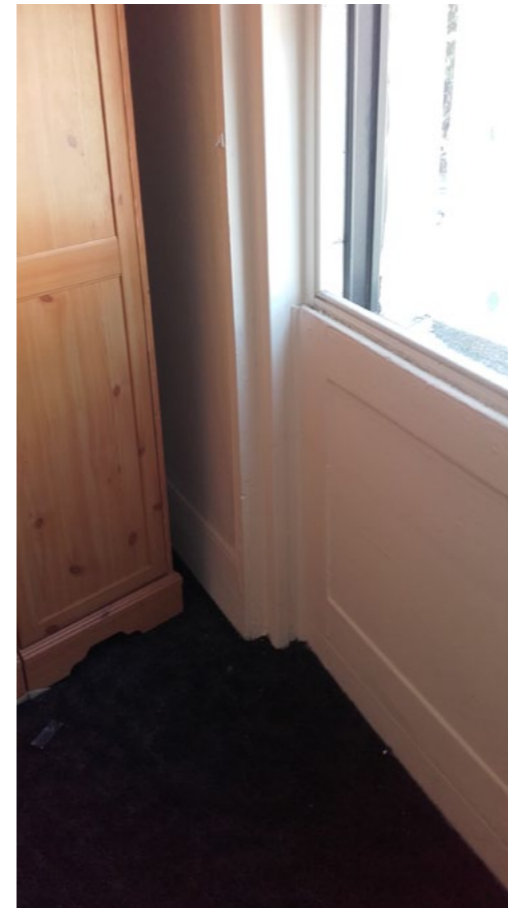
Fig 18. Window panels retained
