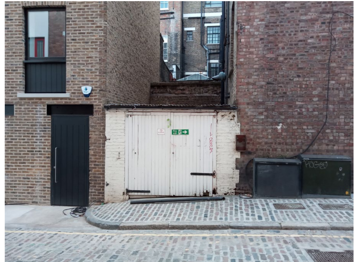
Fig 8. Ext.. Store to be refurbished
