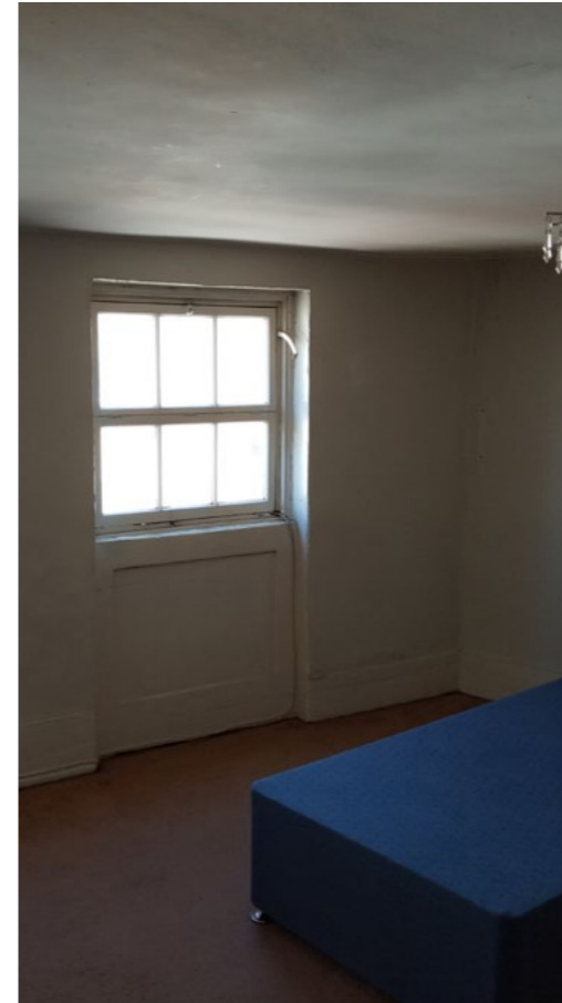
Fig 22. Existing window panels
