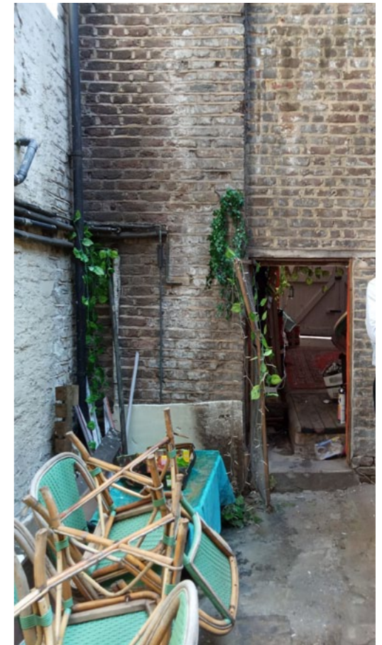
Fig 11. Garage door height increased
