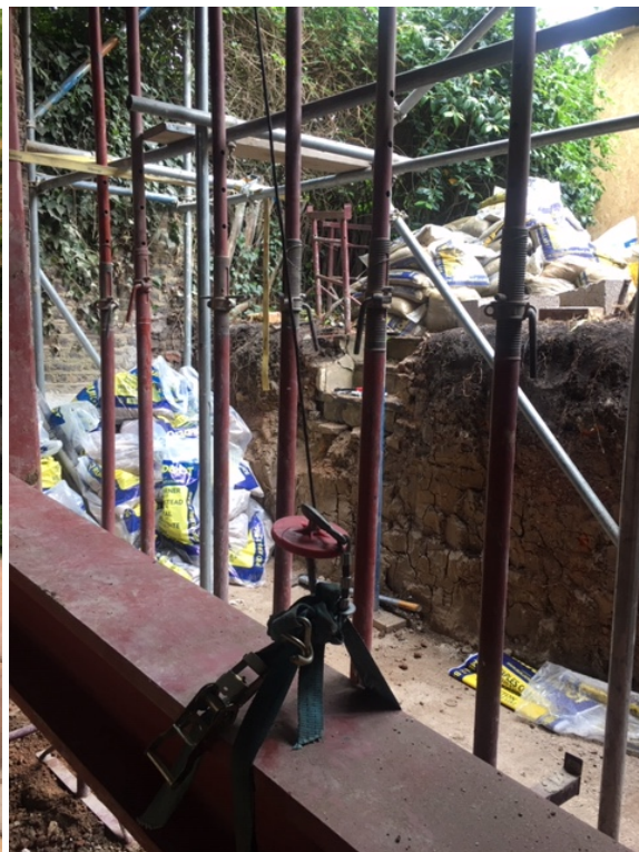
3. Existing rear lightwell area
