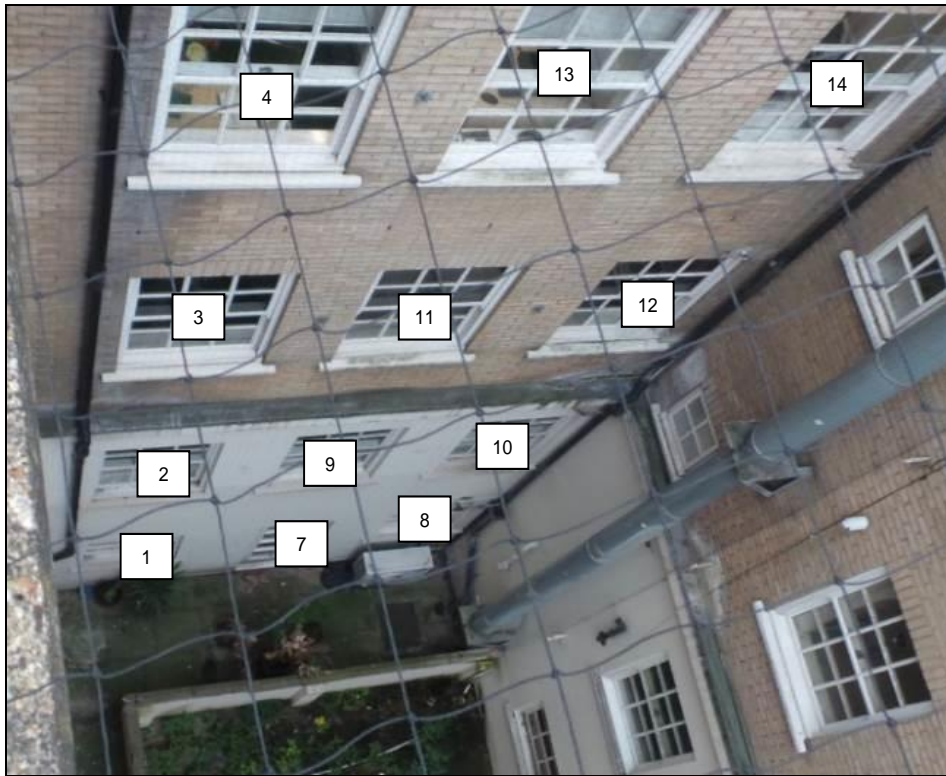
158 to 160 North Gower Street
