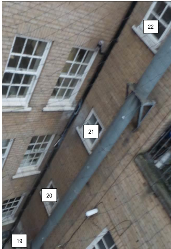
158 to 160 North Gower Street
