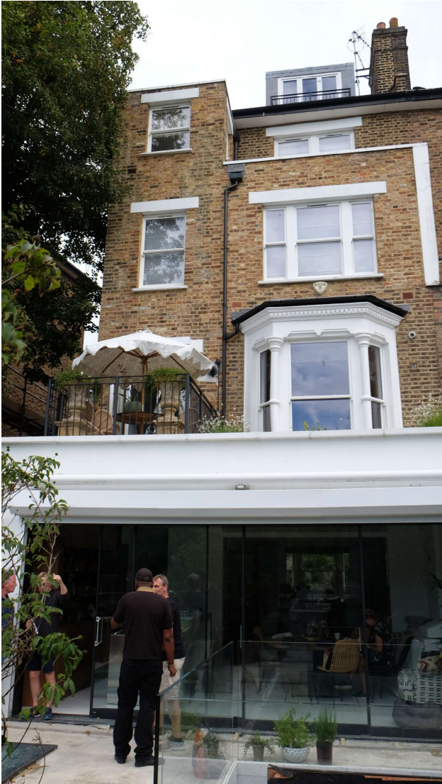
Photo 2 – rear elevation (no. 94).
