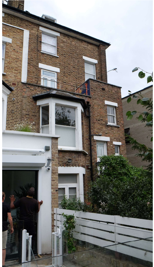
Photo 3 – rear elevation (no. 92).
