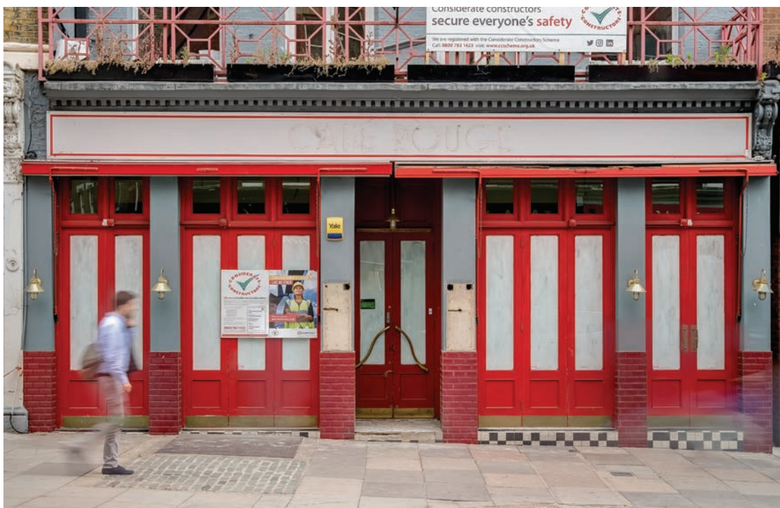
Existing Redundant Dray Hatch Chequer Plate Cover [image source: Author]
