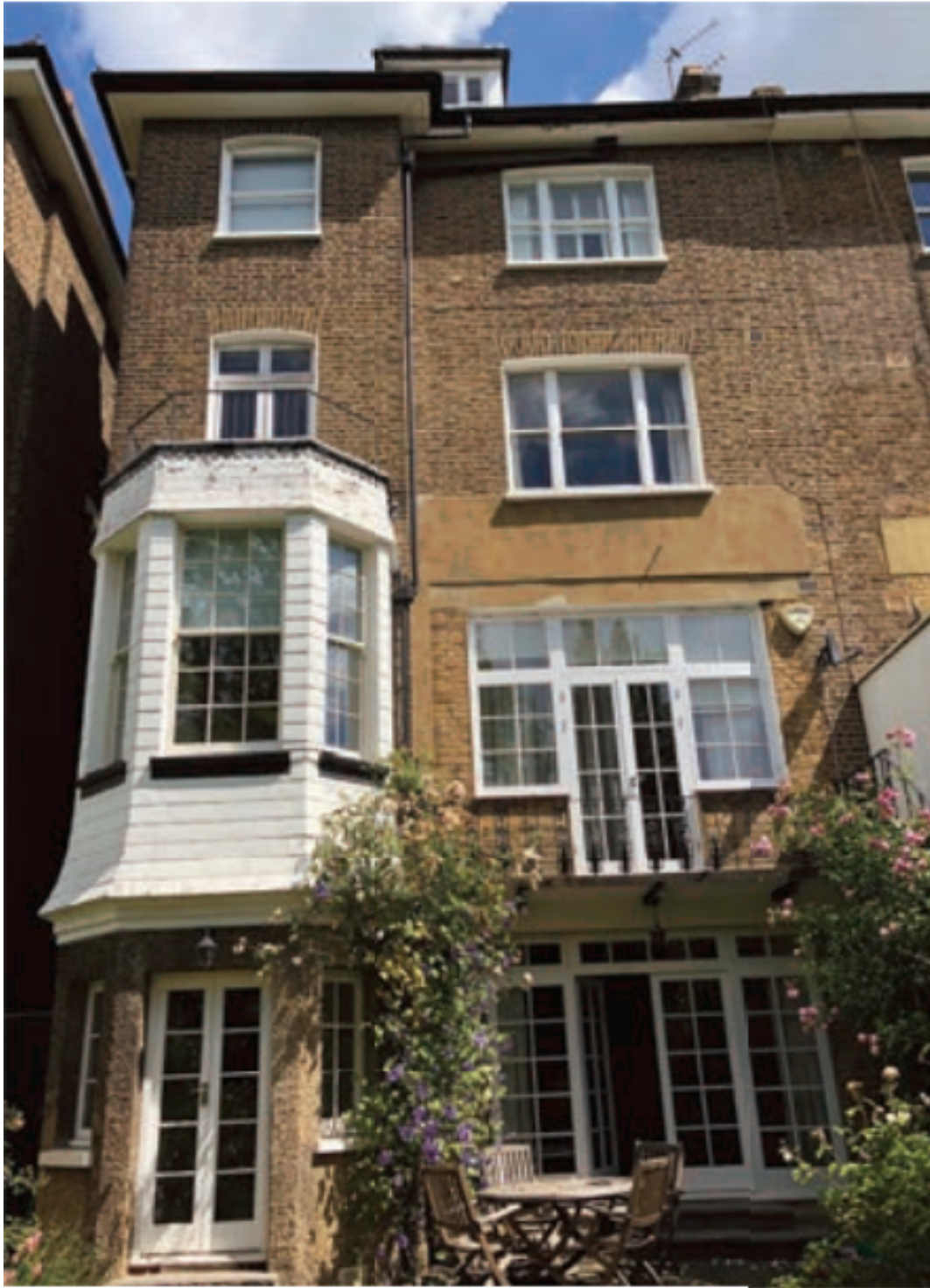
3. Rear elevation of dwelling
