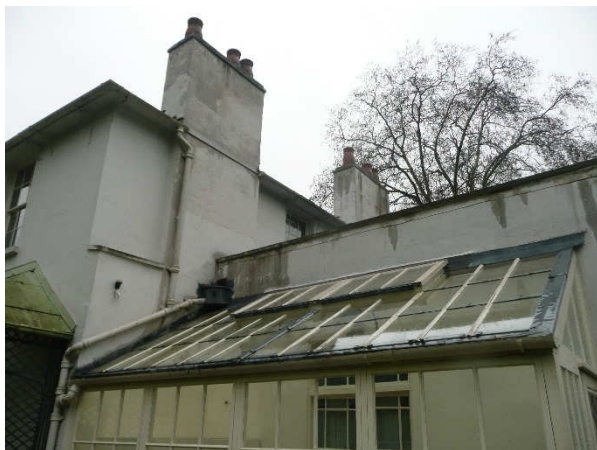
Fig. 7: South Elevation during rain
