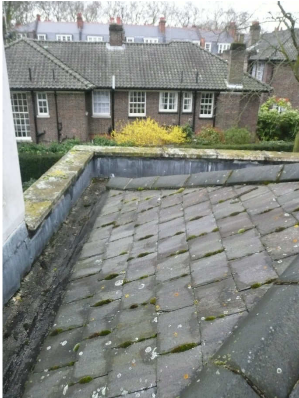
Fig. 9: North East Corner of Annex Parapet
