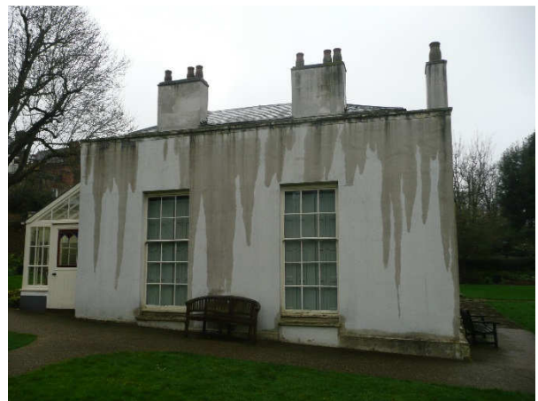
Fig. 6: East Elevation during rain
