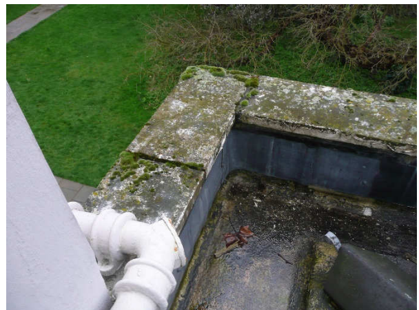
Fig. 8: North West Corner of Annex Parapet
