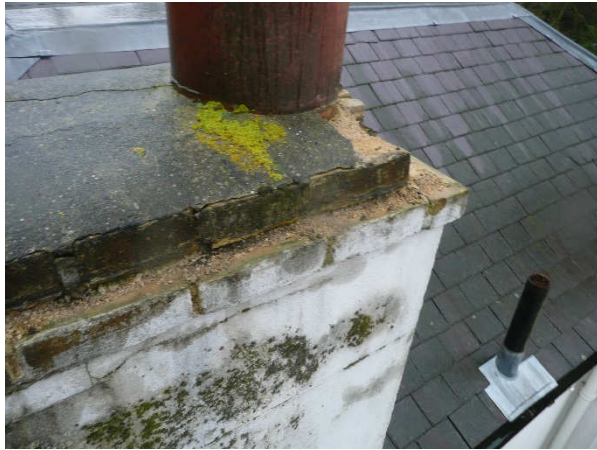
Fig. 17: North West Chimney detail
