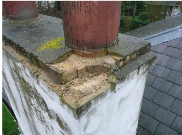
Fig. 18: North West Chimney detail
