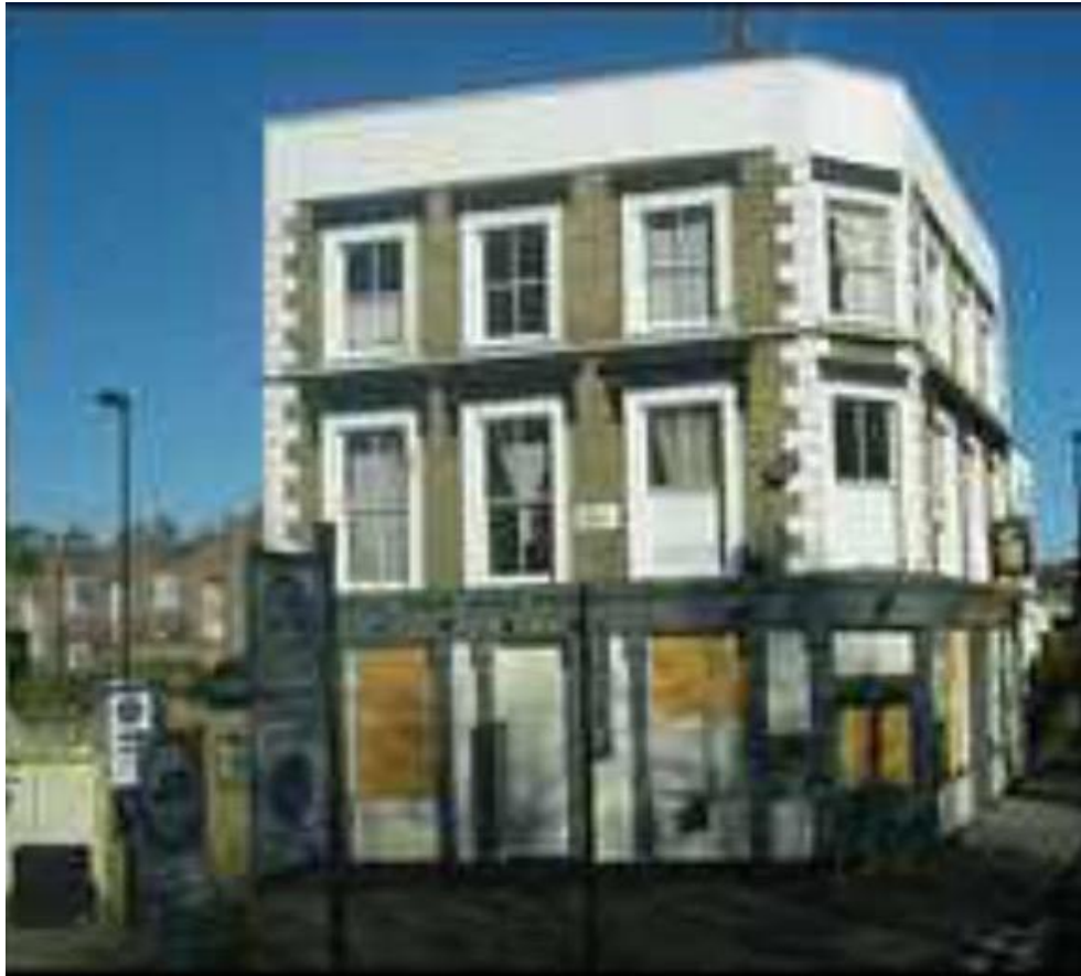
Photograph post closure of The Leighton.
