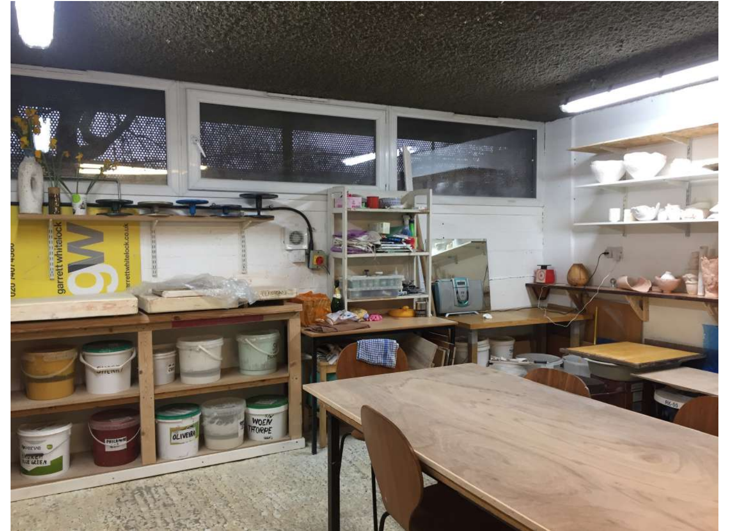
View from inside a ceramic studio at the London School of Mosaic, current tenant of the Ludham Undercroft. Showing windows that have been placed on the inside face of the existing steel grilles.
