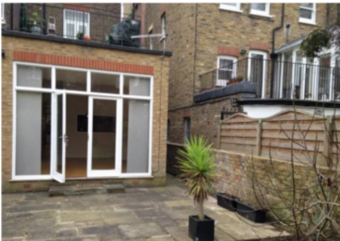
Flat 2 Existing rear window/door (January 2019)
