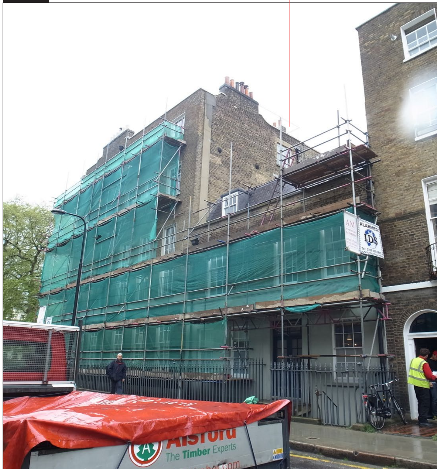
Before (prior to demolition works)
