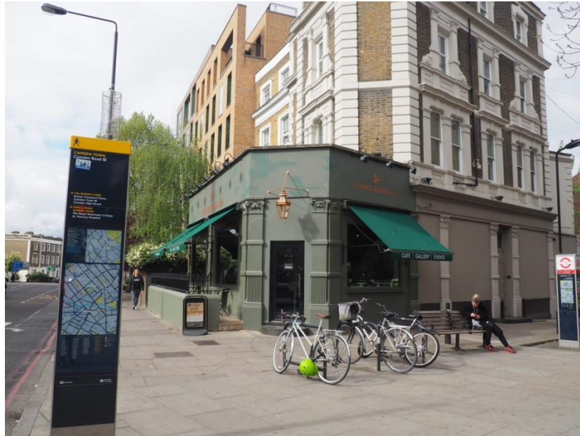
Figure 1 - View of property from Camden Road
