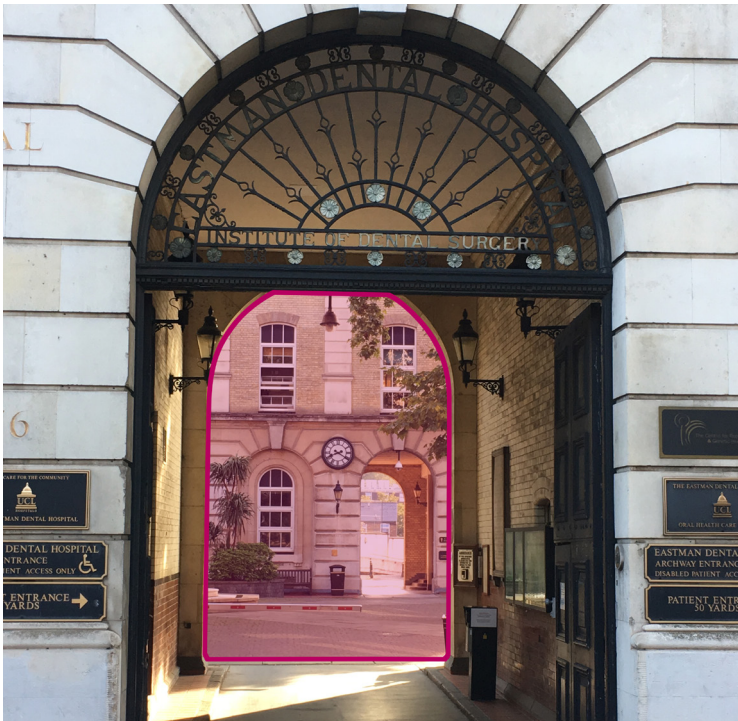
Current view of Courtyard Entrance showing heritage asset loss
