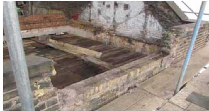
Photo 02 - High level parapet to the south facade to be raised to match existing.
