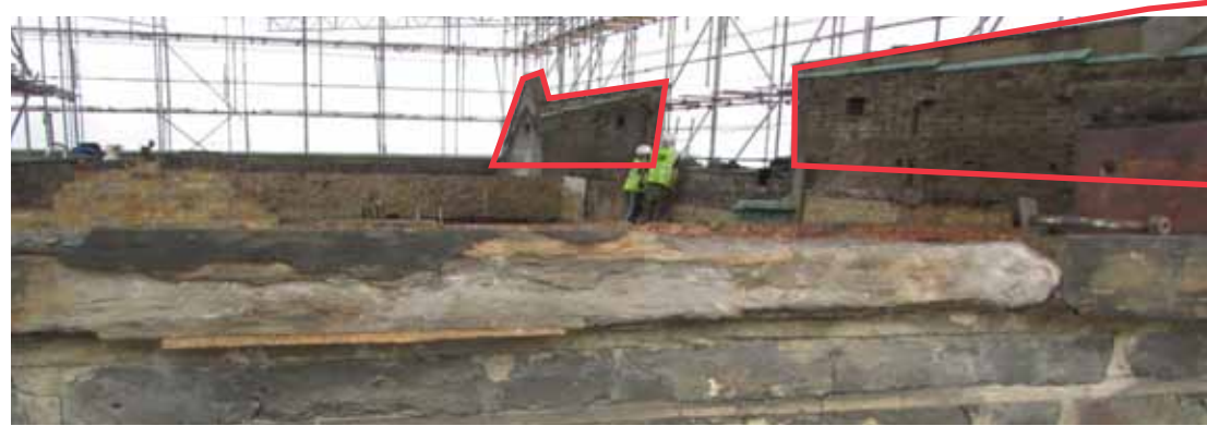
Photo 01 - Existing high level parapet wall to be lowered to match existing parapet level to south, north & west facades. The above photo shows the existing York stone copings are largely degraded on the sky surface. Virtually all the copings are delaminating laterally along bedding planes leaving the whole unit friable.
