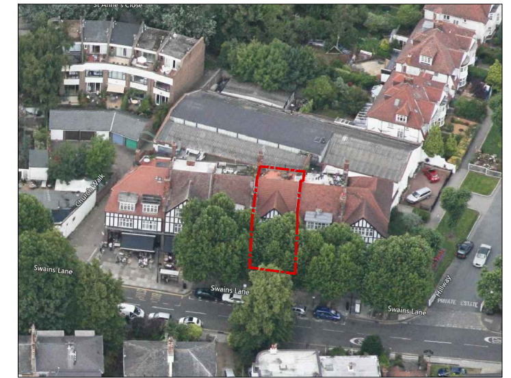
Aerial view of South Elevation
