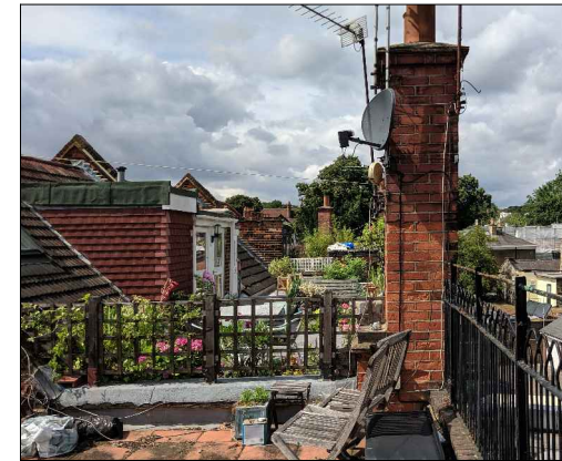
Roof terrace and rear dormer to residential unit at no. 19C Swain's Lane
