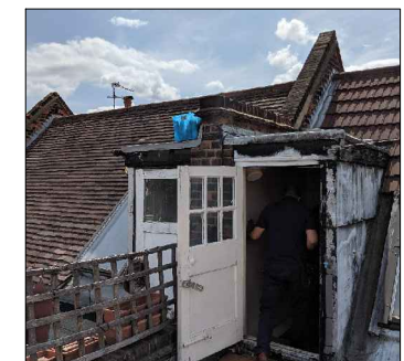
Roof access at no. 21B Swain's Lane
