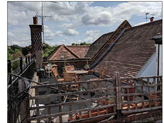
Roof terrace to residential unit at no. 23 Swain's Lane
