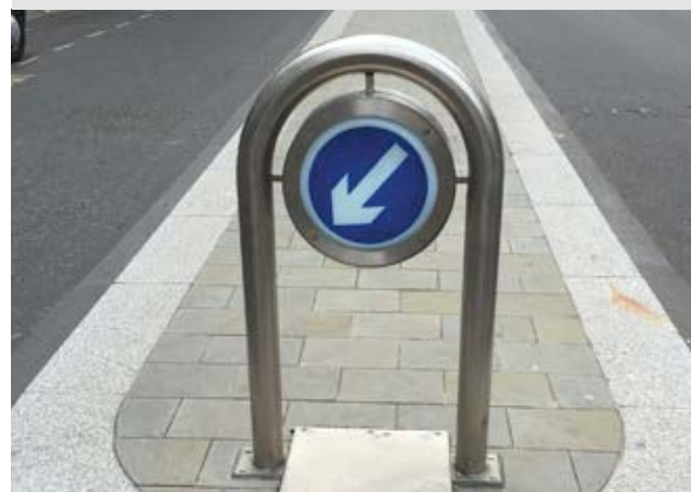
Figure 213: A 'keep-left' hoop bollard which is internally illuminated
