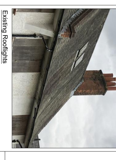
lead aprons to lower edge. - Cast Iron framed, single glazed rooflights with
