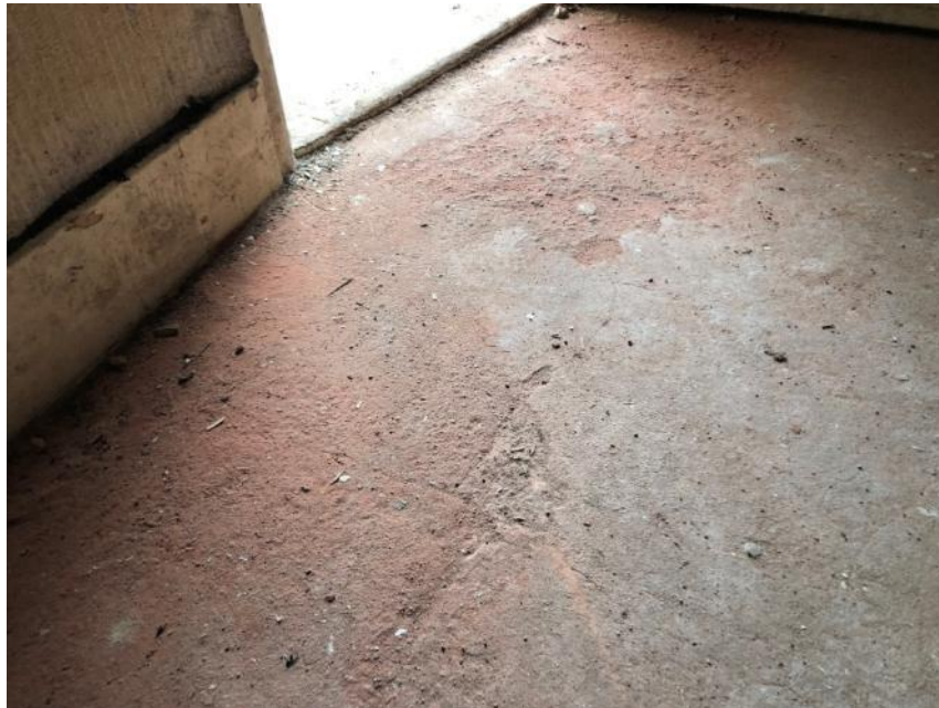
Surface abrasion adjacent to entrance door
