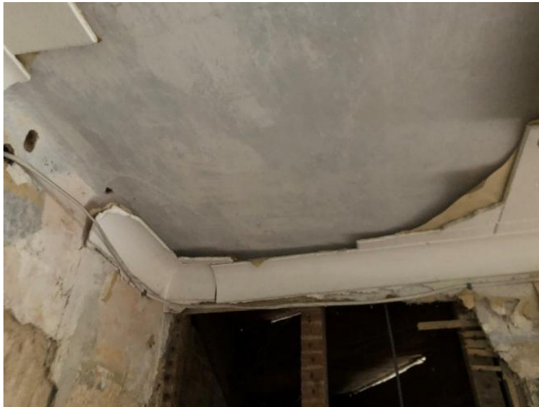
De-bonded polystyrene tiles and covings
