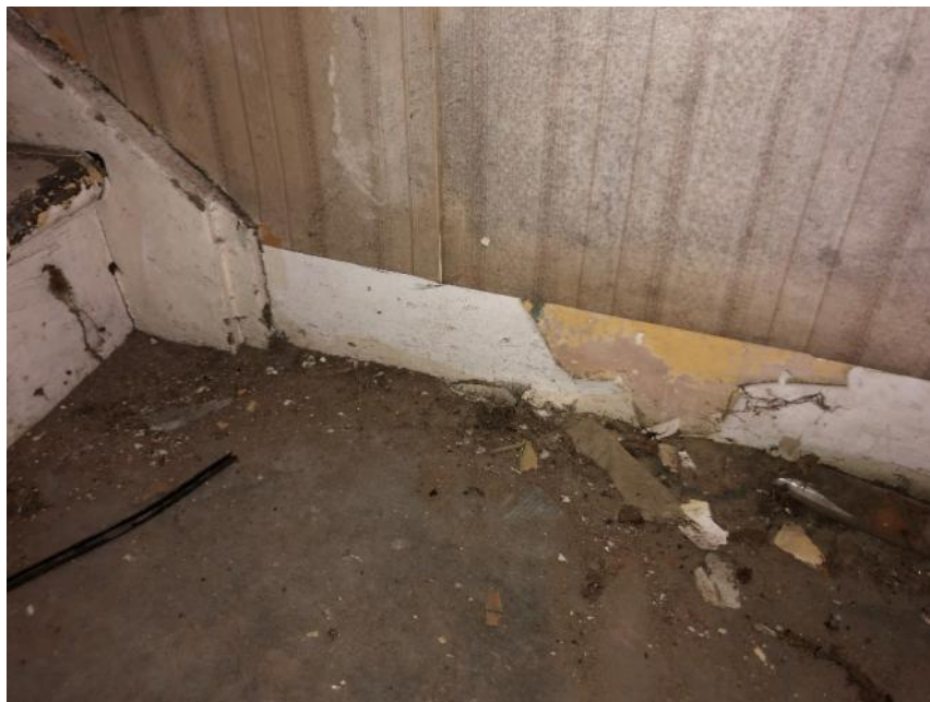
No skirtings fitted to north wall
