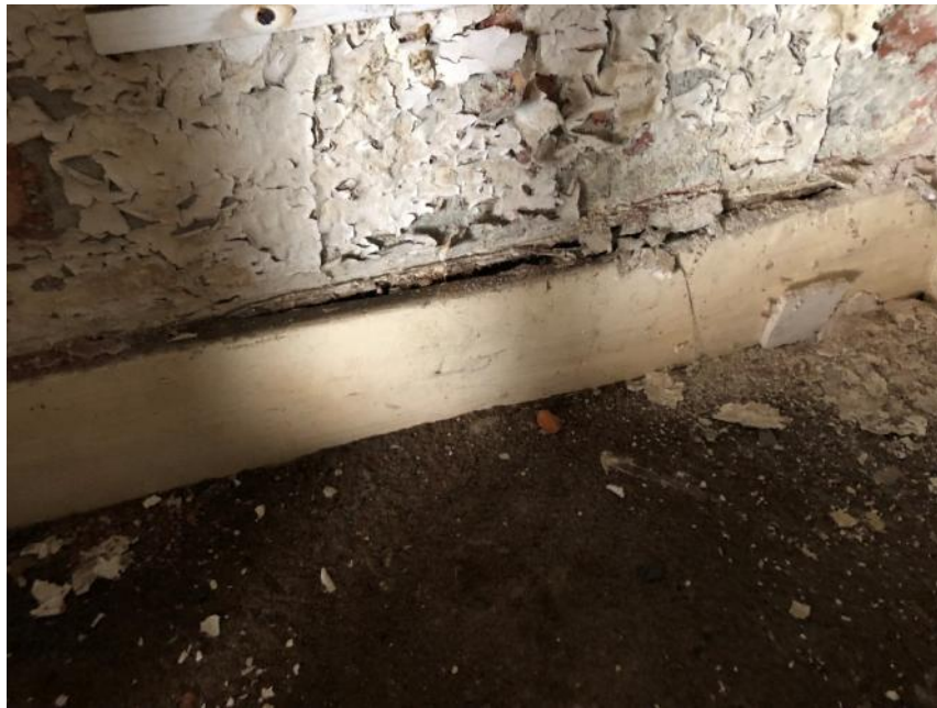
Damp affected wall surfaces to south-west corner
