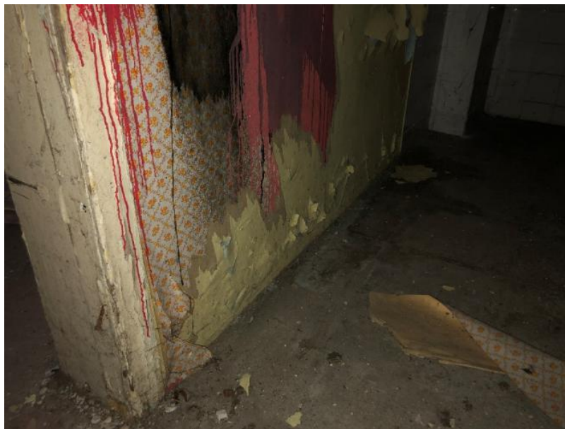
Damp affected wall surfaces
