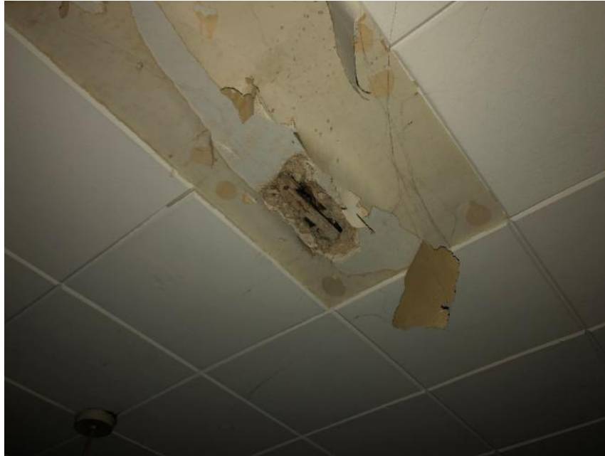
Damaged plasterwork
