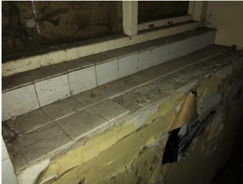
Damage caused by the removal of former wall mounted fittings
