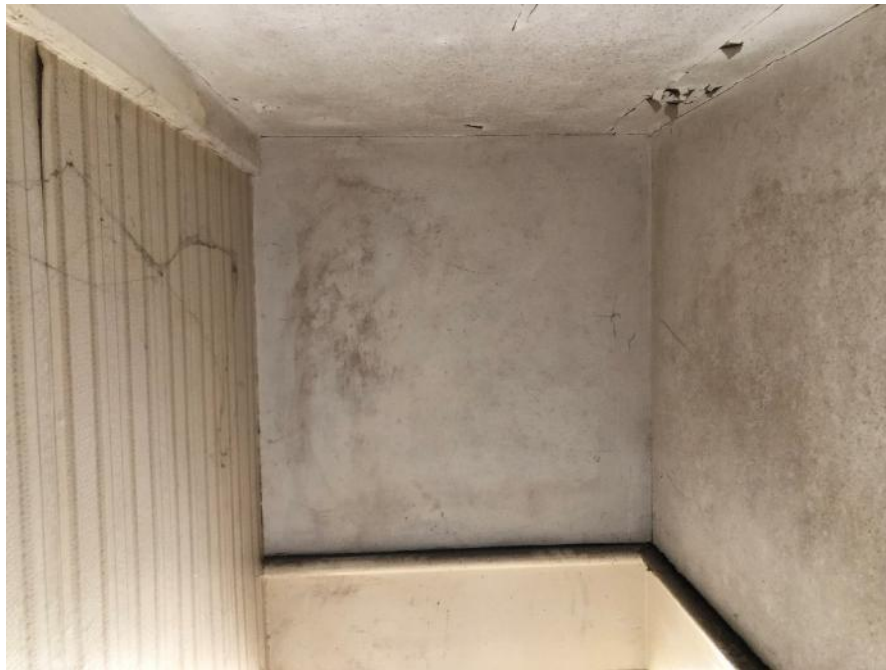
Overboarded timber panelled landing walls
