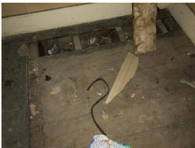
1 no. timber floorboard removed
