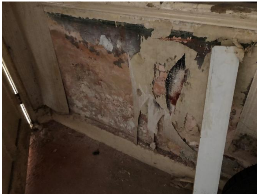
Damp affected wall surfaces to east wall
