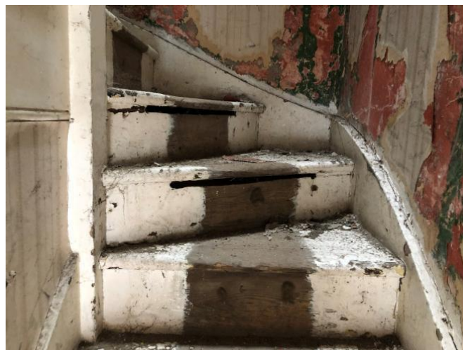
Stair winders to first floor landing
