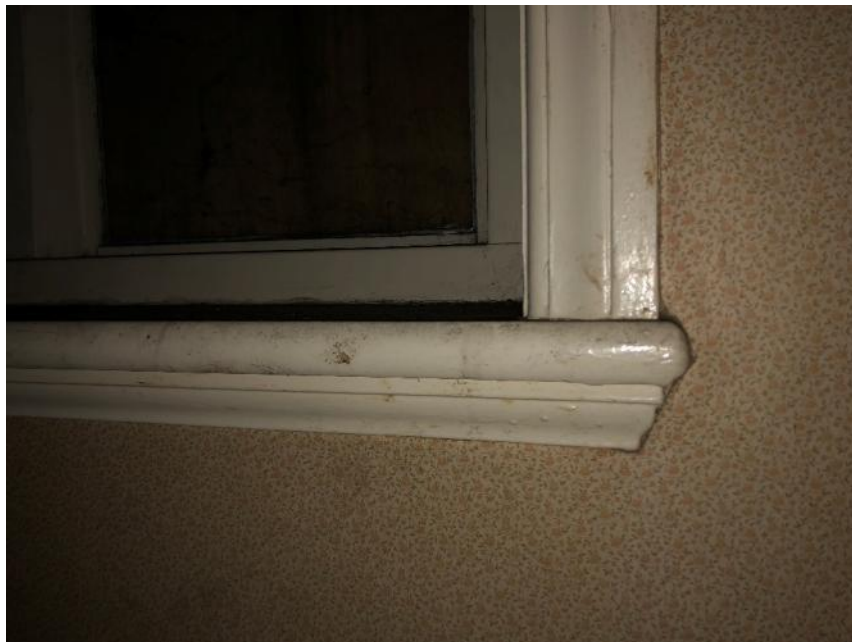
View of existing window board and beading
