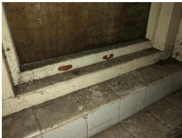
View of opening unit and ceramic tiled cill
