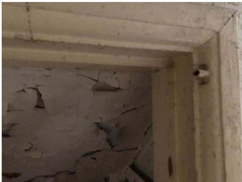
Door lining and architrave detail
