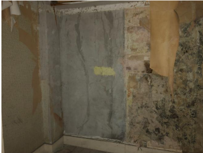
View of former chimneybreast position
