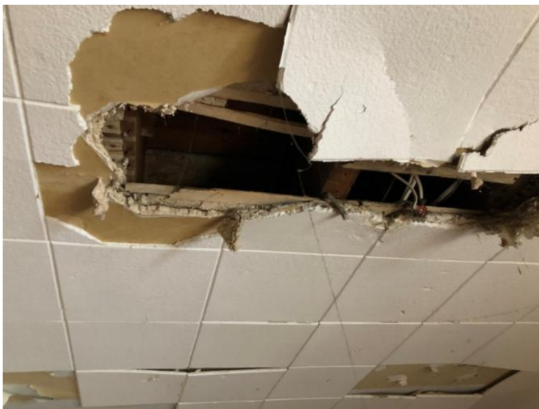
Damaged polystyrene tiles and plasterwork
