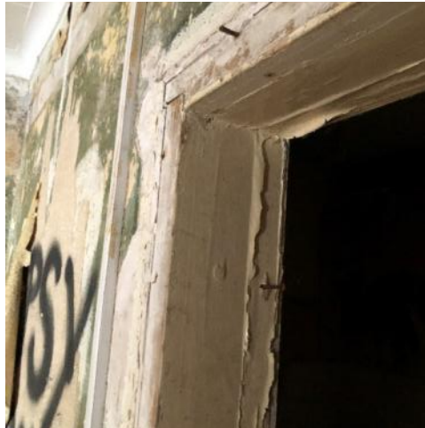
Damaged lining and architrave to Kitchen entrance
