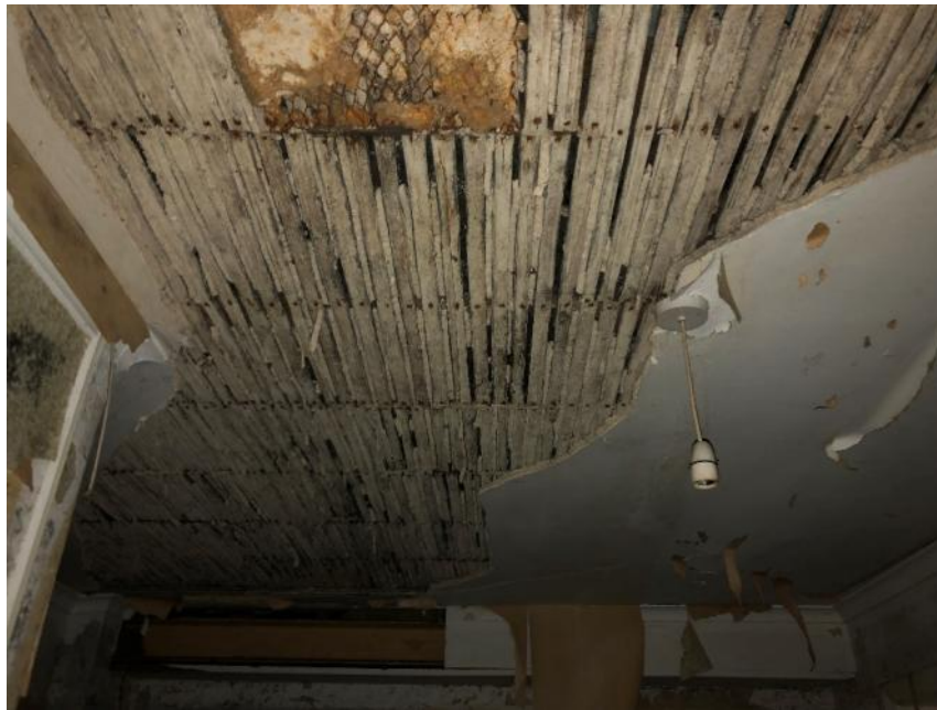
Collapsed area of bedroom ceiling
