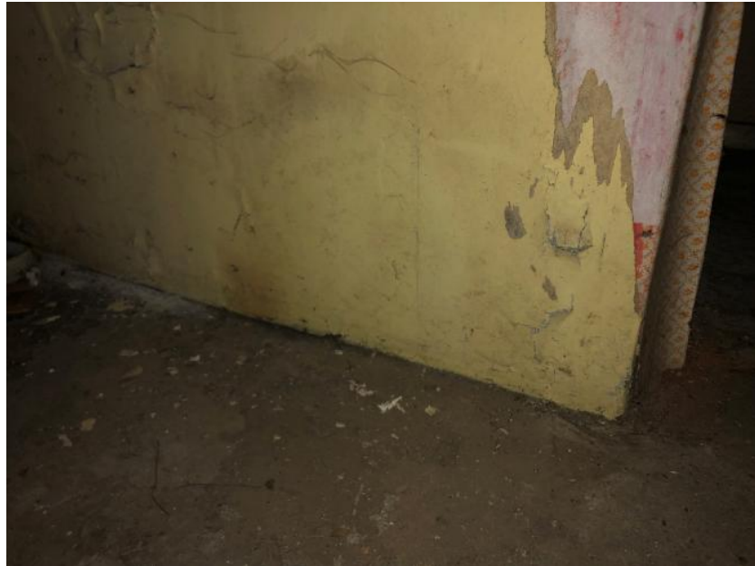
No skirting boards installed
