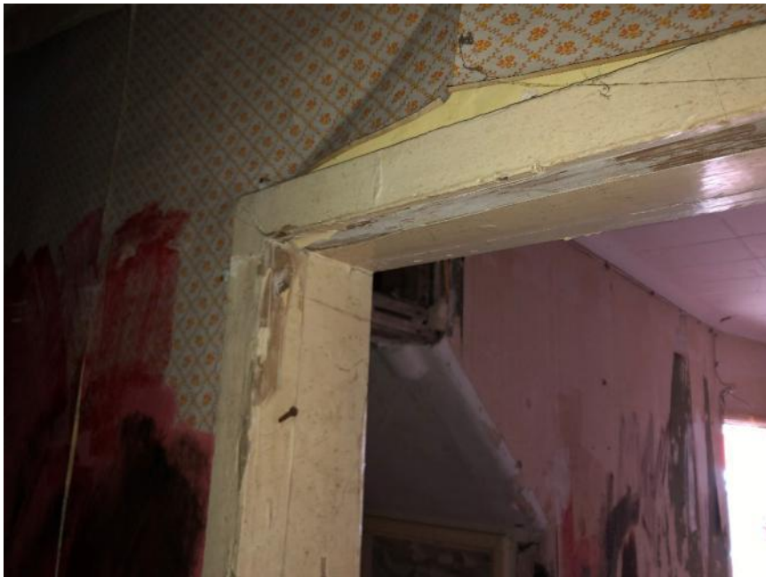
Decayed timber door lining and architrave
