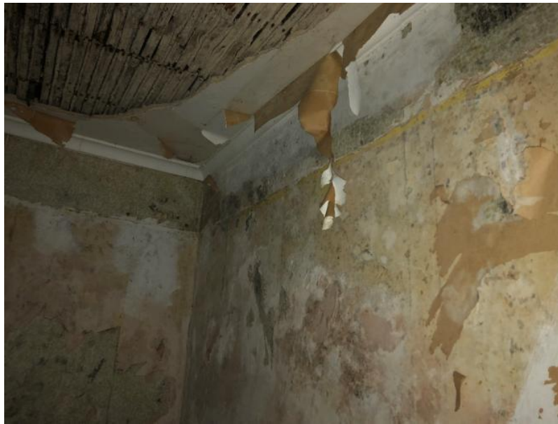
Damp affected and damaged plaster surfaces
