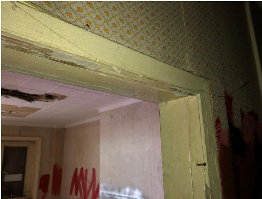
Door lining and architrave to kitchen entrance
