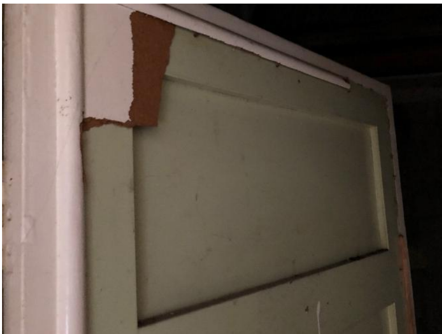
Damaged plywood overboarding to Bedroom 2 Entrance door
