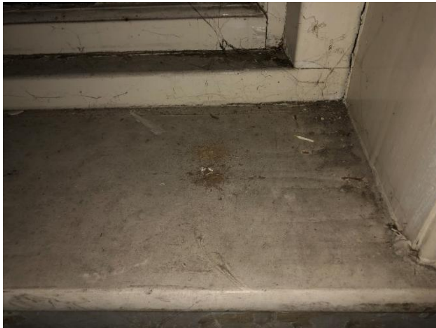
View of damaged timber window board
