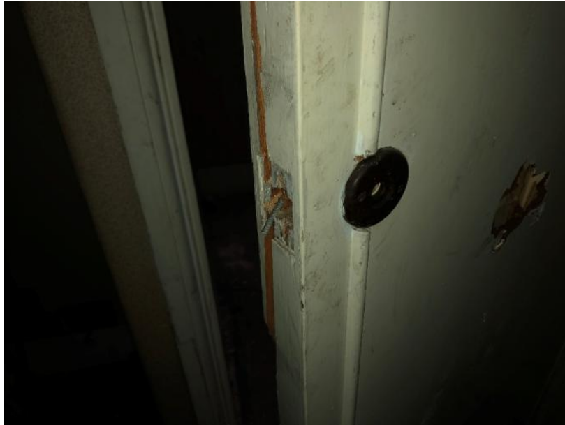
Damaged/missing plastic door furniture to Bedroom 1
