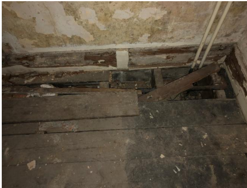
1 no. lifted timber floor board
