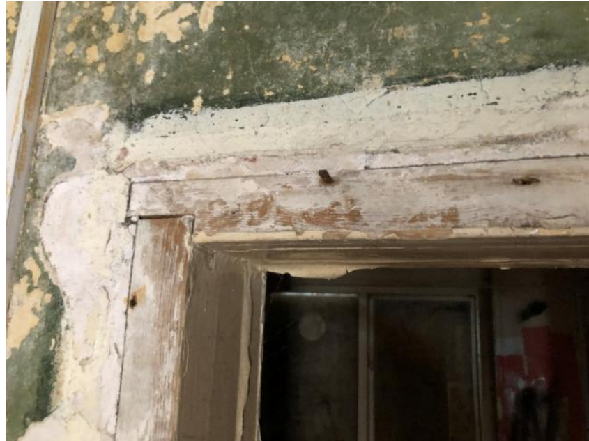
Missing door architrave detail
