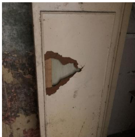
Damage to overboarded surface
