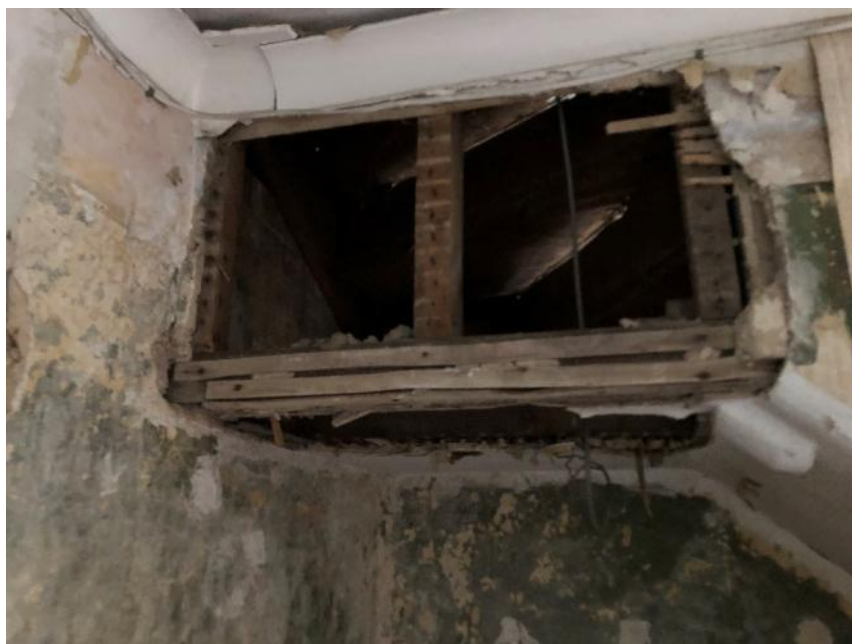
Damaged and damp affected plaster surfaces at high level
