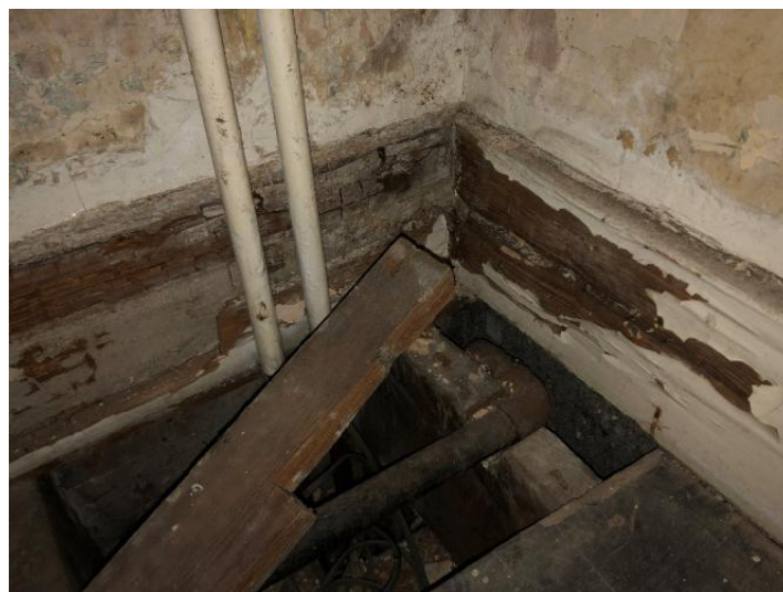
View of decayed skirting boards
