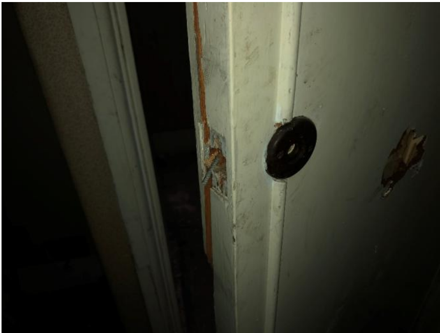
Split/damaged timber to leading edge of Bedroom 1 entrance door
