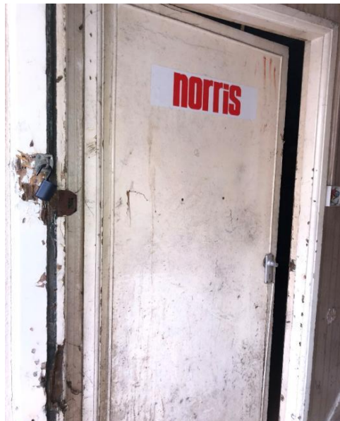
Overboarding to external face of door
