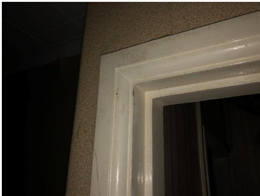
View of entrance door lining and architrave
