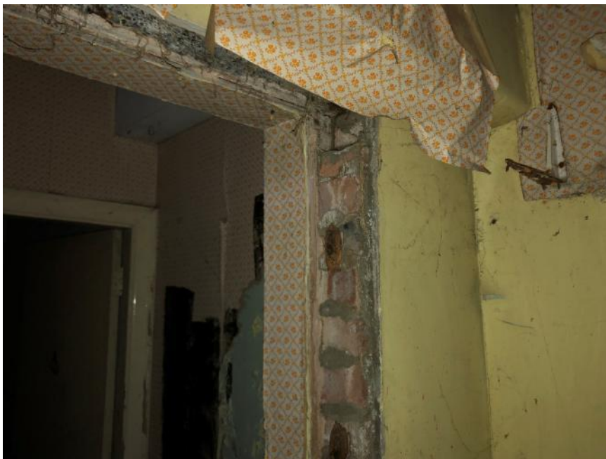
Door lining and architrave to rear entrance lobby removed
