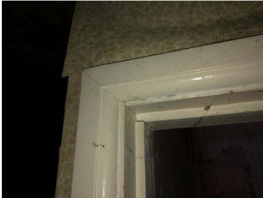
View of entrance door lining and architrave
