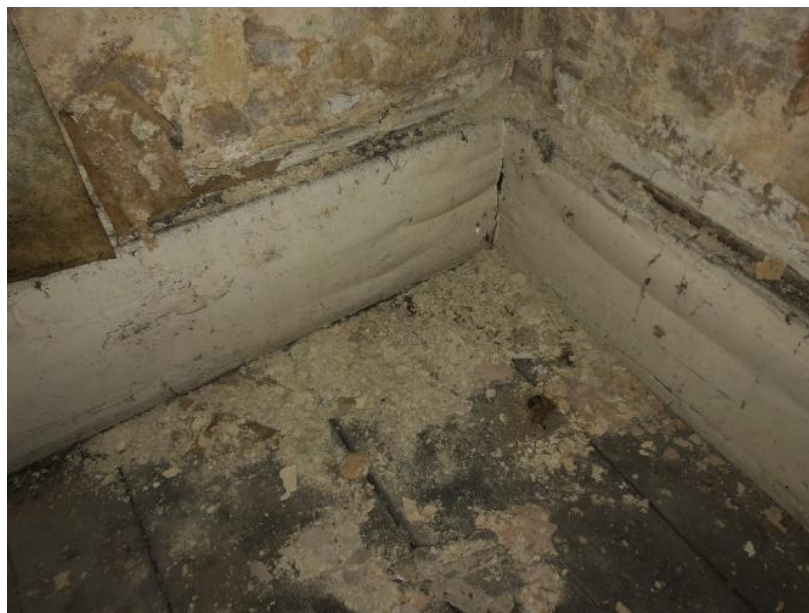
Damp affected plaster surfaces
