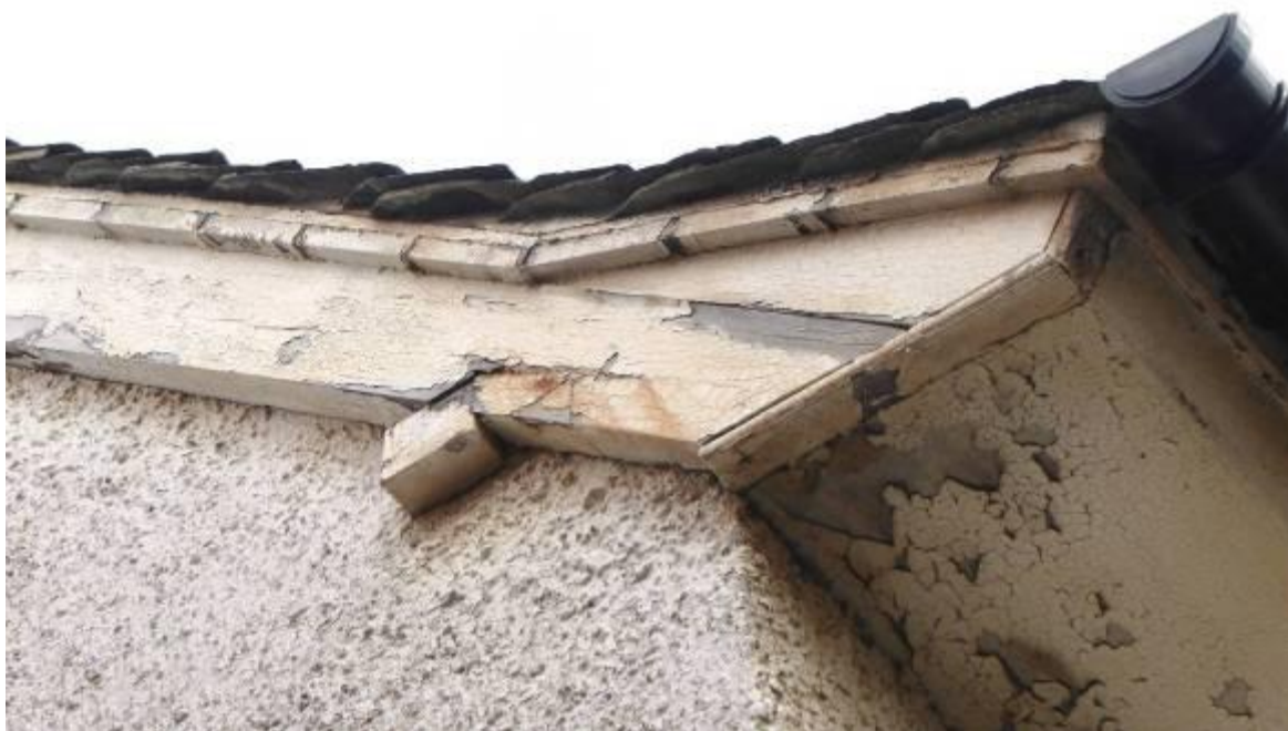
Fig 3.3.1: Main roof eaves and gable junction
