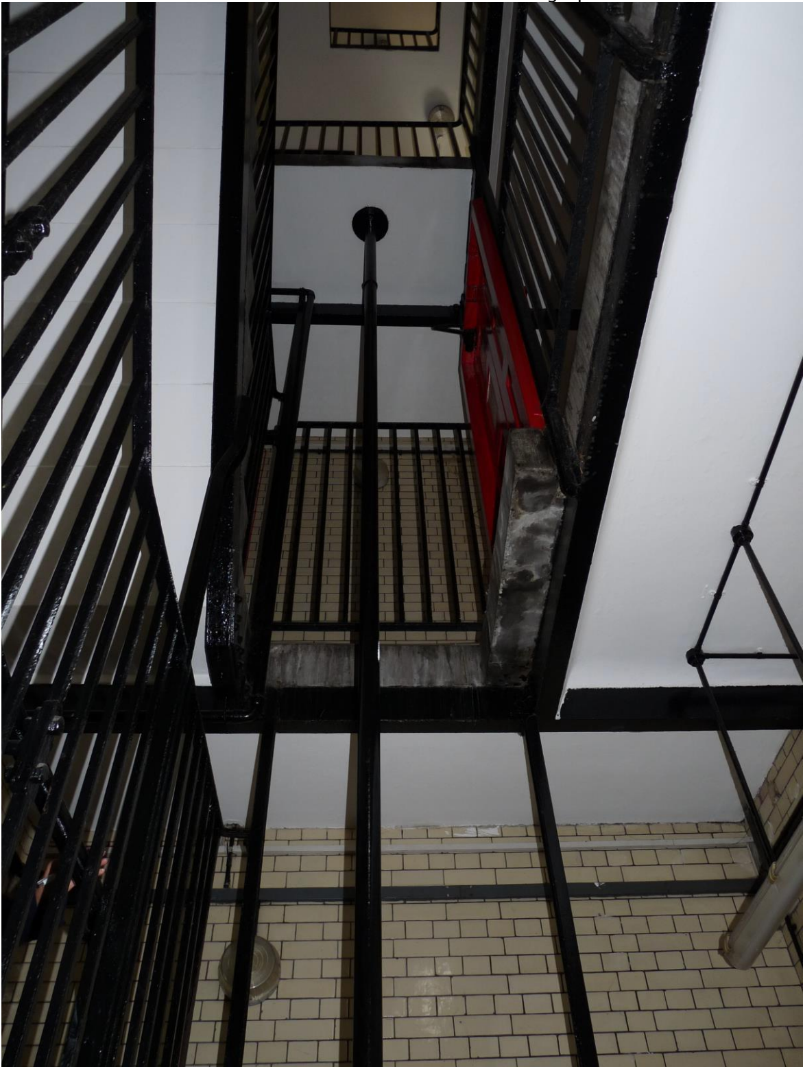
Photograph of stair tower interior
