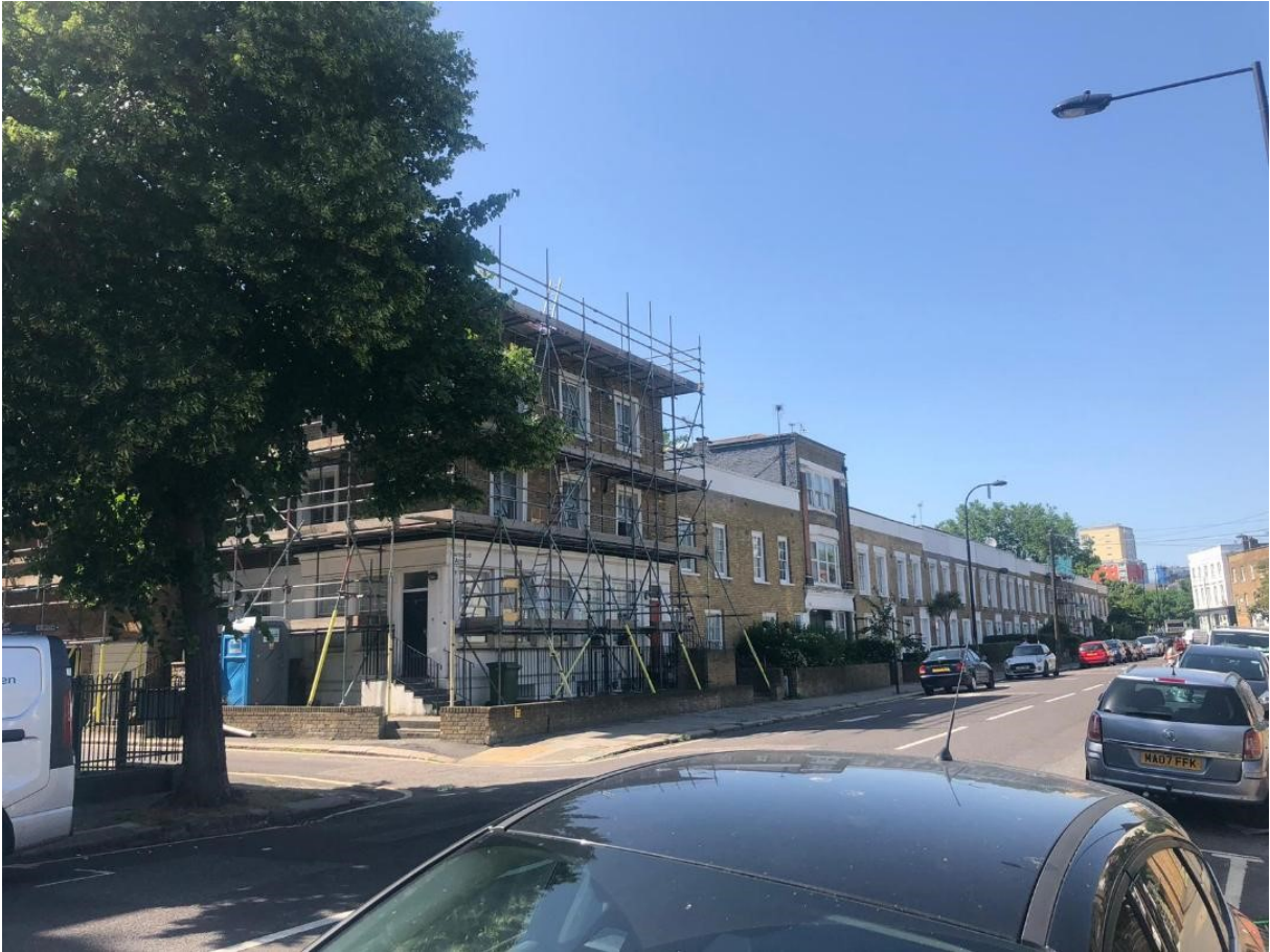
Harmood Street, Street View, looking towards Prince of Wales Road
