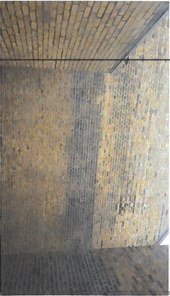
existing view to the rear of No. 12 Hatton Wall
