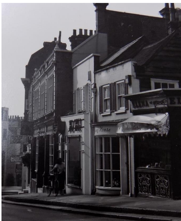
View of September 1981, showing the new shopfront of 1956 with central doors flanked by bow windows with small panes, some with bull's eyes (P.D. Barkshire, Camden Archives, acc. no. 033354)
