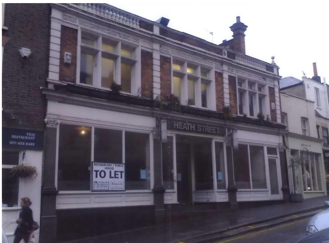
2008 view of the Heath Street elevation, showing the shopfront installed by Bass for All Bar One in 1998-9 (App. No. LK9802243R3 / P9802242R3).
