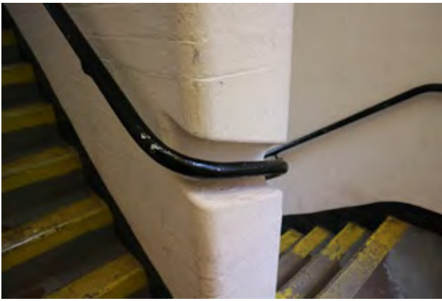
66. Stairwell showing cut-away for handrail, Panther House (Insall, 2018)
