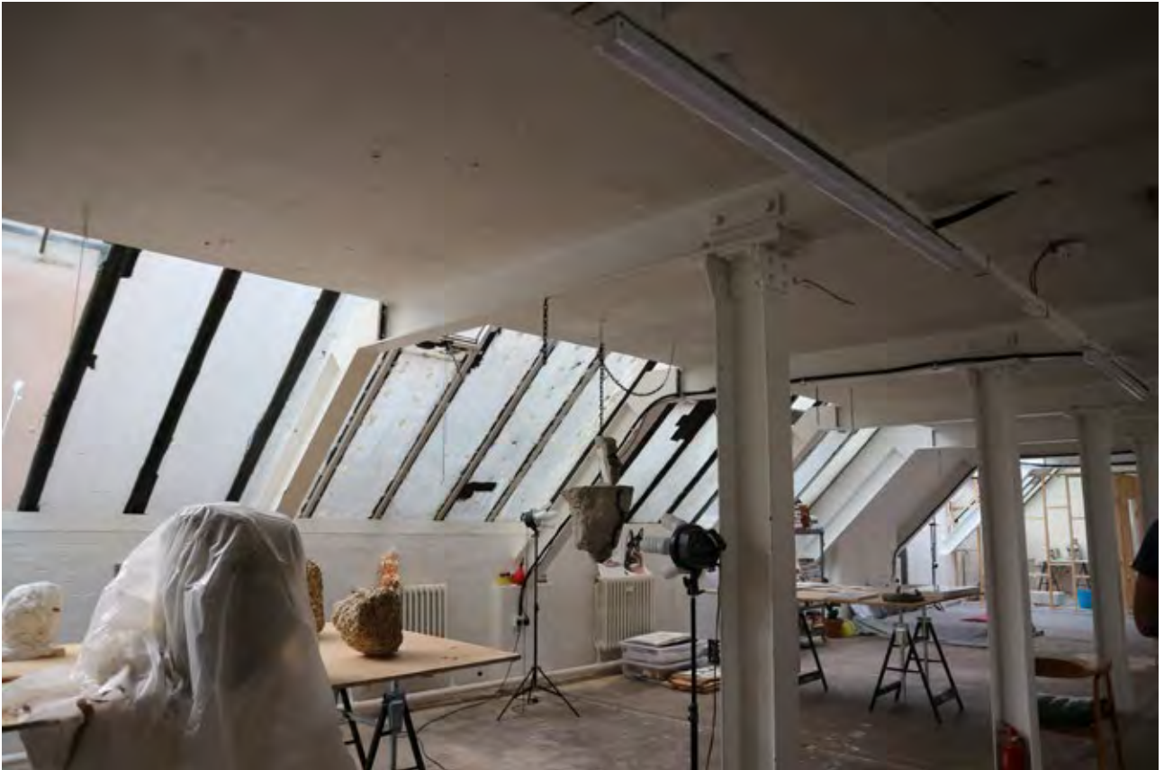
76. Second floor level of Block C (Insall, 2018)
