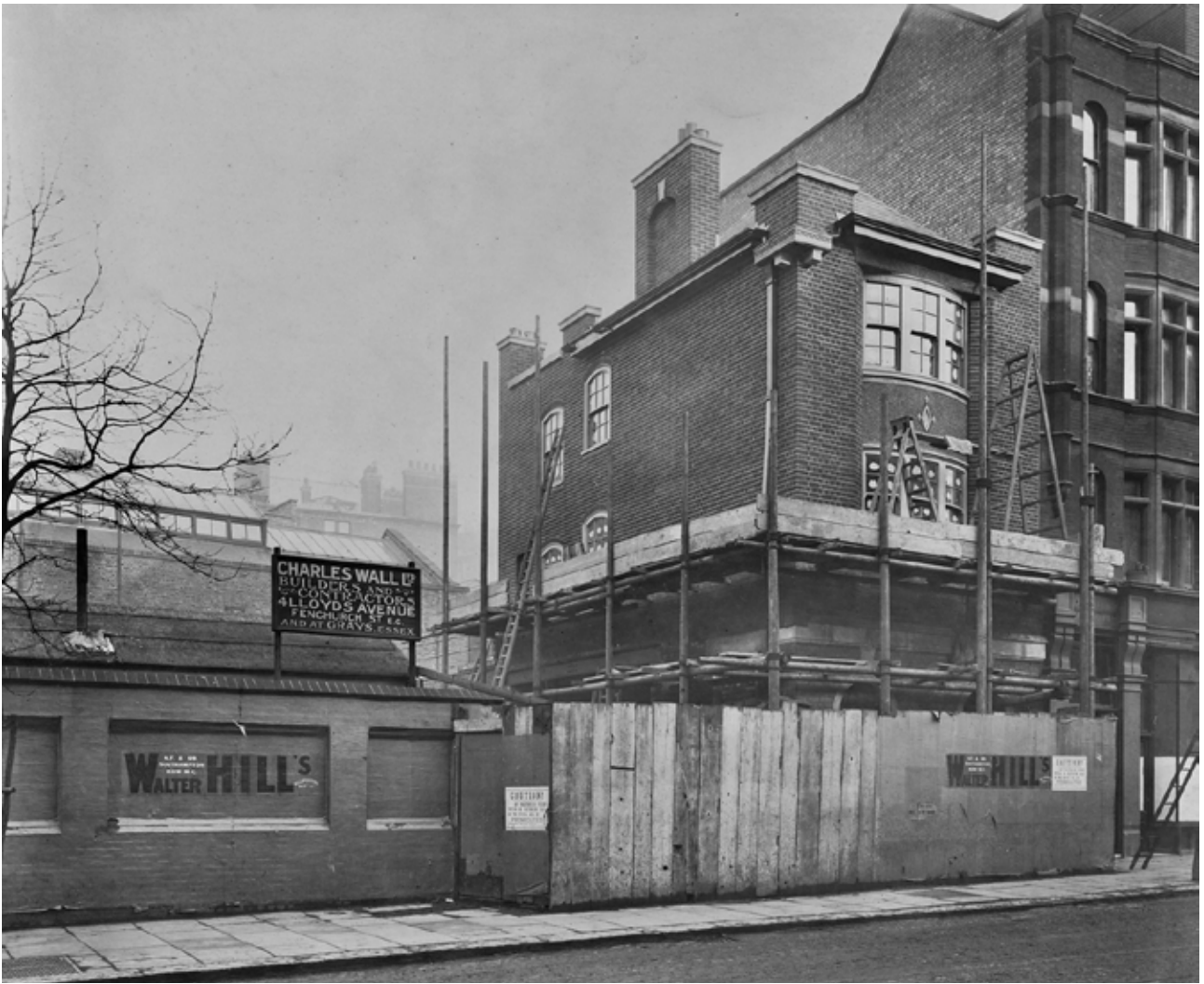
41. Exterior of the foreman's house at 156-158 Gray's Inn Road, 1907 (Collage)
