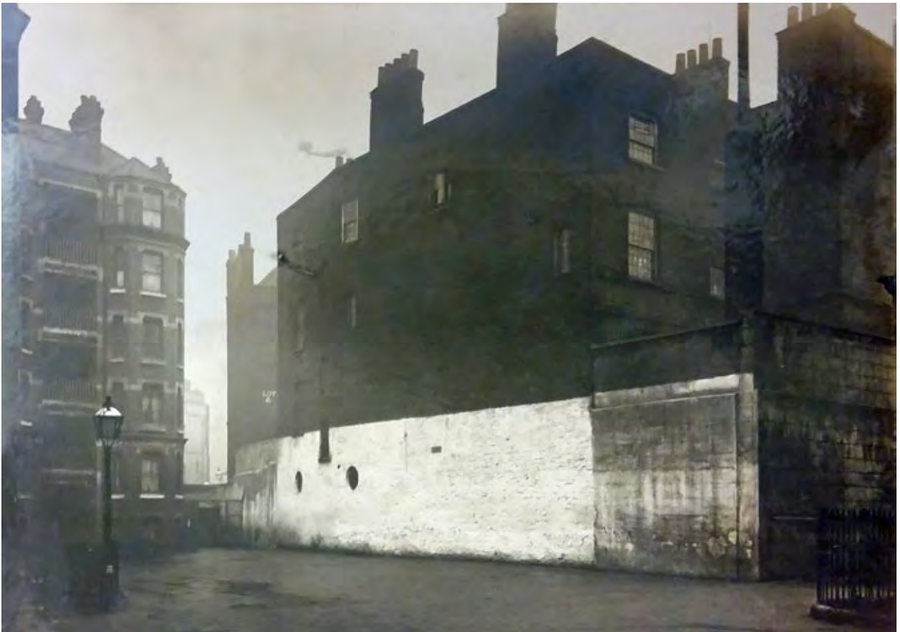
12. Holborn Union Workhouse showing the north exterior wall between the site and the newly built Holsworthy Square ,c.1888(Camden Archives)
