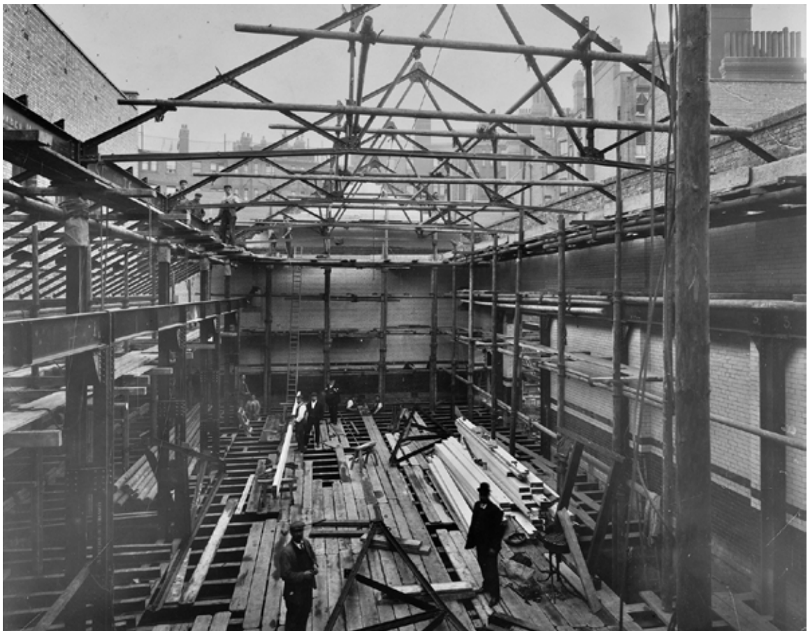
31. Holborn substation during construction, 1906 (Collage)
