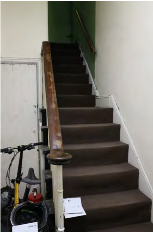
85. Ground floor staircase of the house at 156-158 Gray's Inn Road (Insall, 2018)
