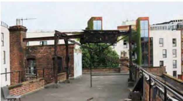
60. Roof of Block A showing 1950s electric hoist (Insall, 2018)
