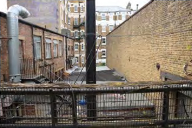
89. 160-164 Gray's Inn Road rear elevation (Insall, 2018)
