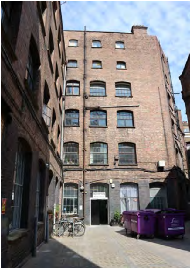
61. Panther House Block B South elevation (Insall, 2018)
