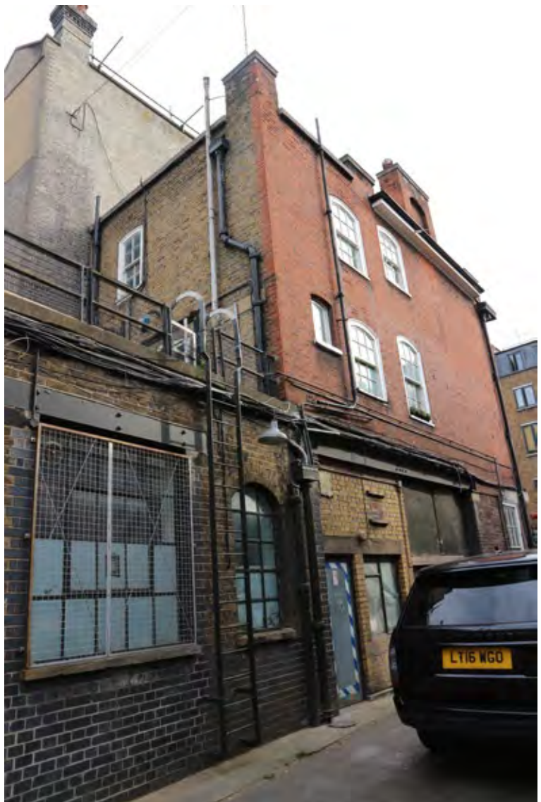
82. 156-158 Gray's Inn Road yard showing side and rear elevation of Foreman's house (Insall, 2018)
