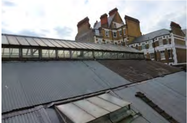
79. Roof of the former substation (Insall, 2018)
