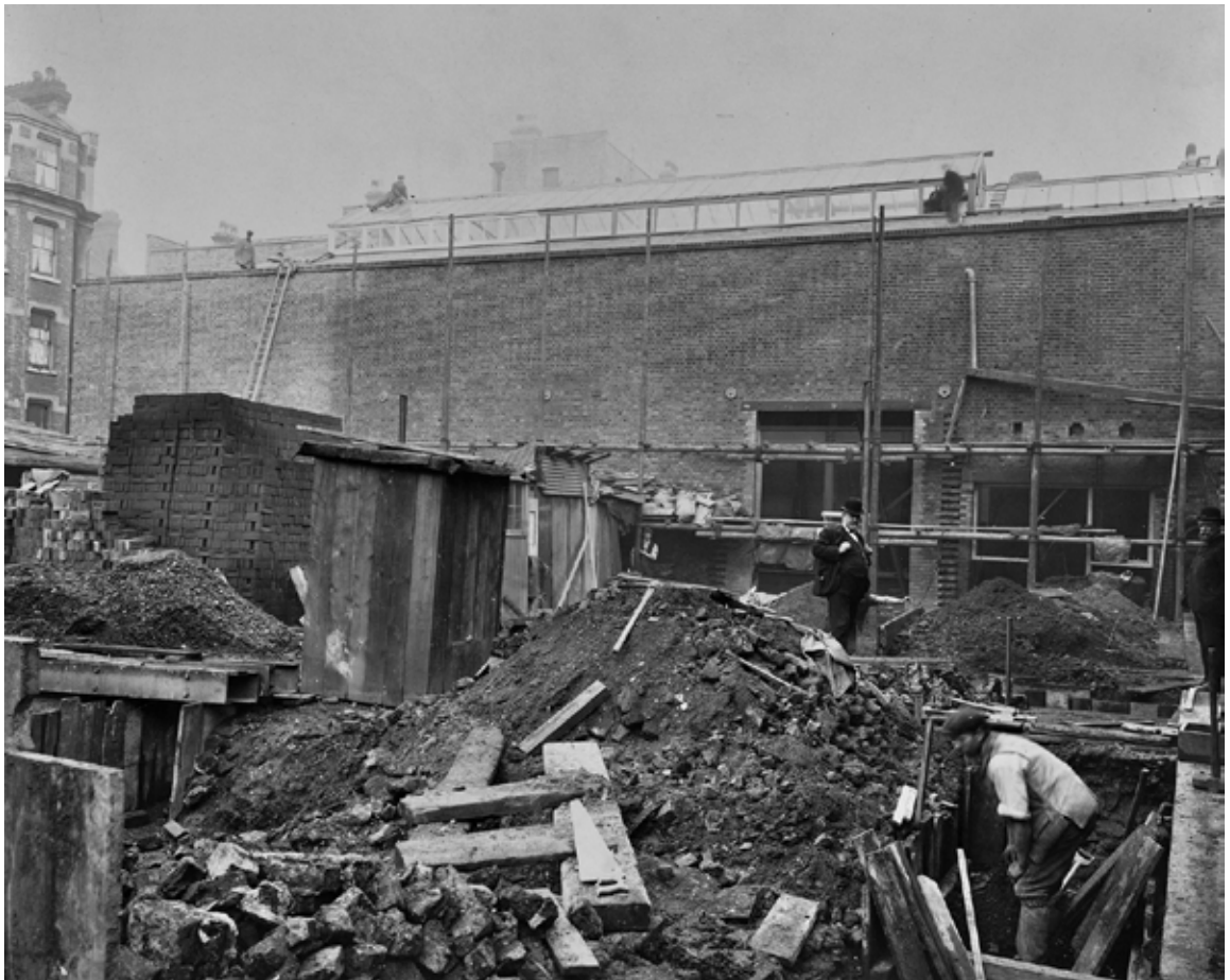
30. Holborn substation during construction showing the construction of the mess, 1906 (Collage)
