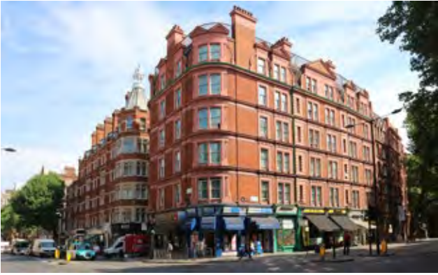
50. Dawlish Mansions, Gray's Inn Road and Gray's Inn Buildings, Rosebery Avenue (Insall, 2018)
