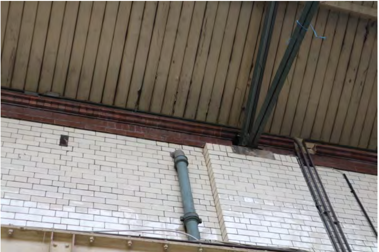
84. Detail of the cornice (Insall, 2018)
