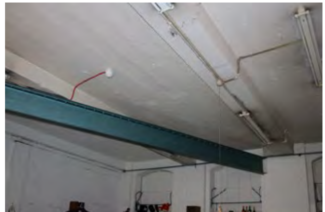
72. Gantry, ground floor Block A (Insall, 2018)
