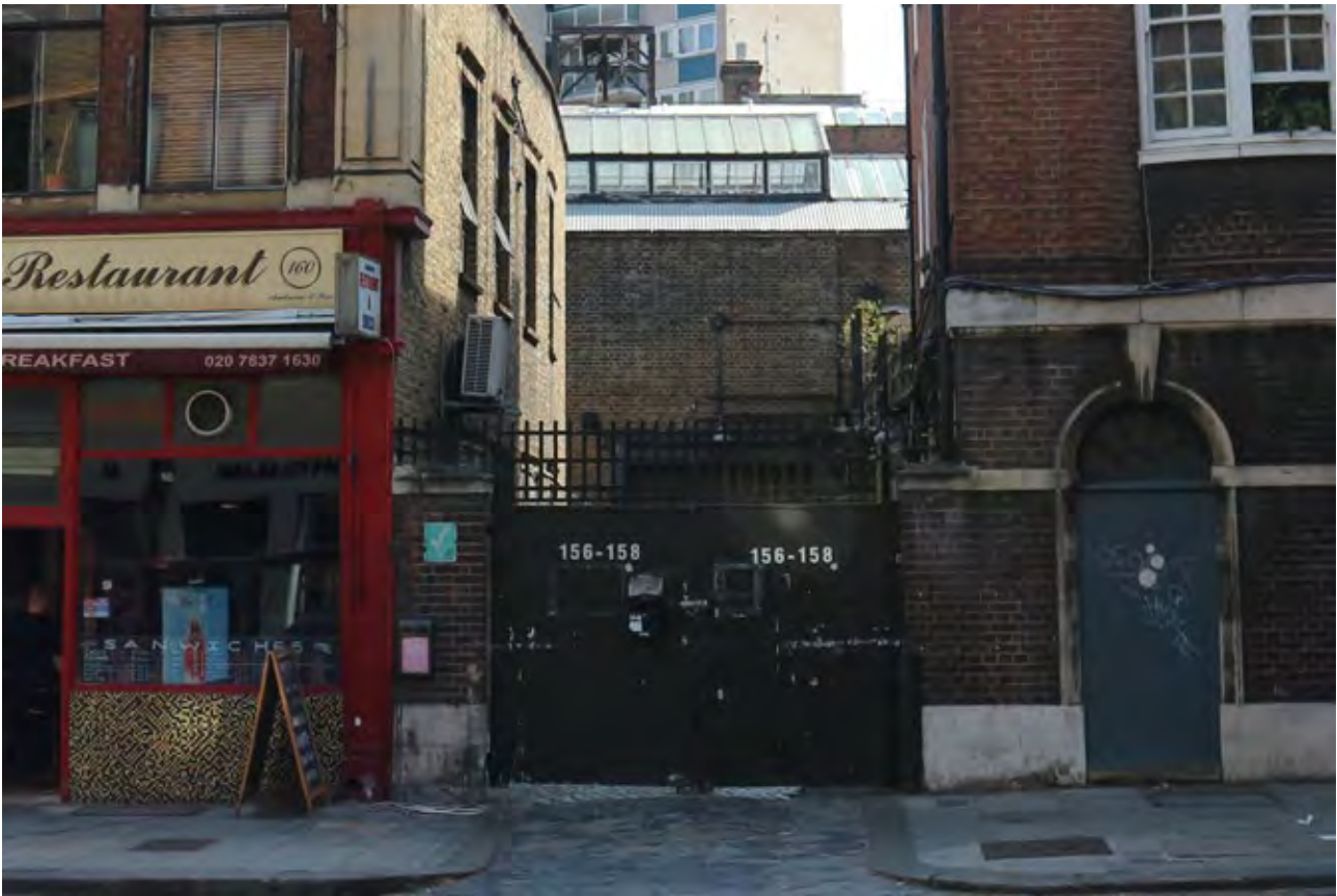
77. Entrance gates to the substation area, 156-158 Gray's Inn Road (Insall, 2018)
