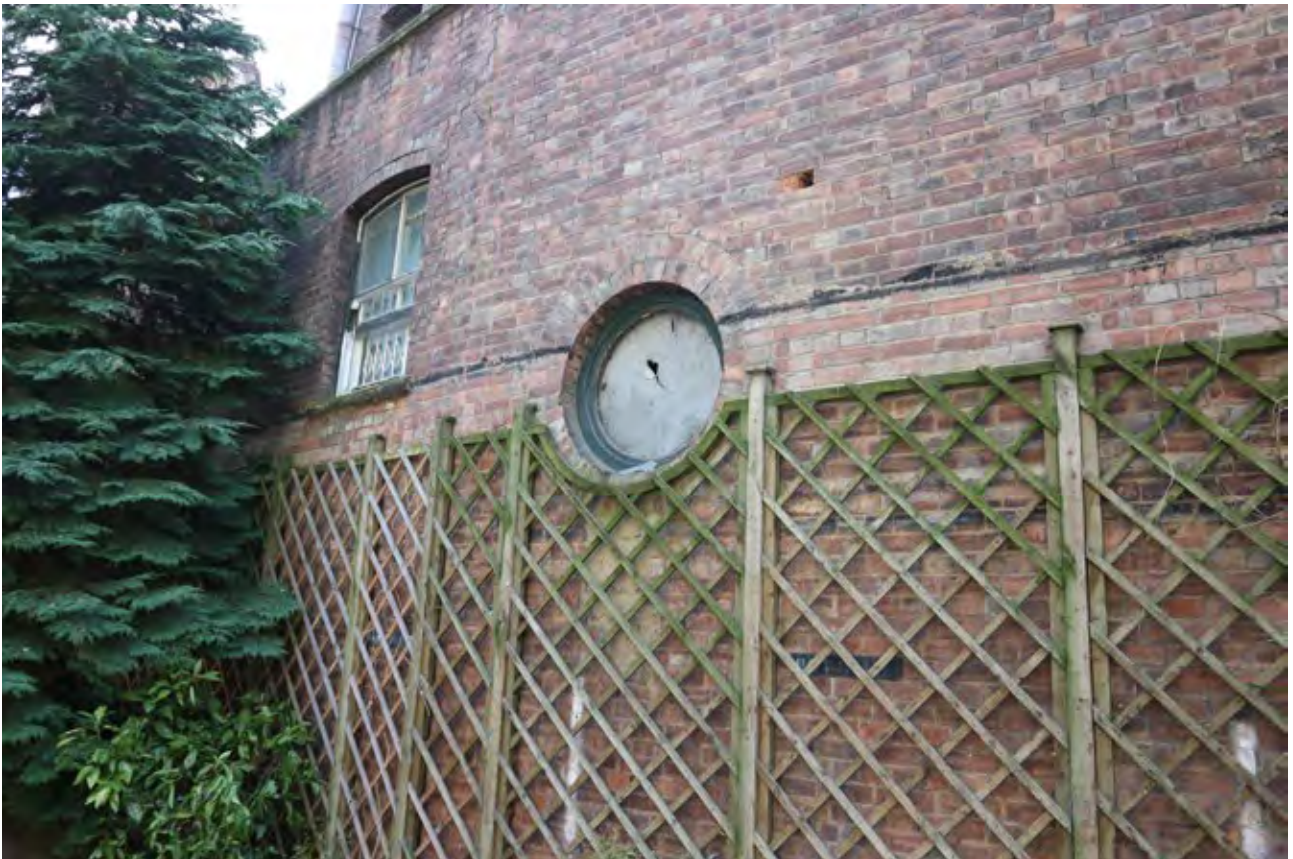
13. North exterior wall of Panther House with porthole and cambered arched window in the same place as Plate 12 (Insall, 2018)
