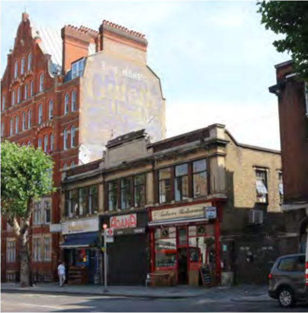
87. Front elevation of 160-164 Gray's Inn Road (Insall, 2018)
