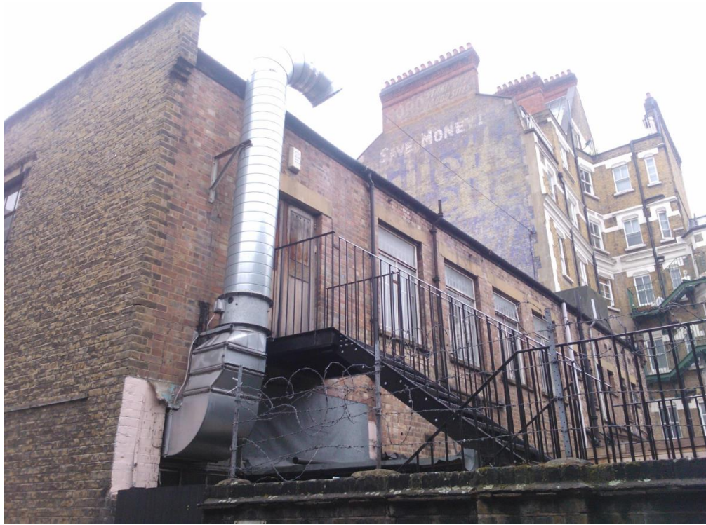
Photograph 7 – Rear view of 160-164 Grays Inn Road
