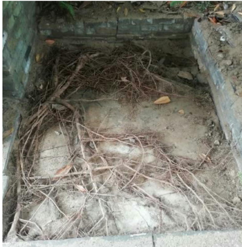
Photograph 1: Roots above vault roof
