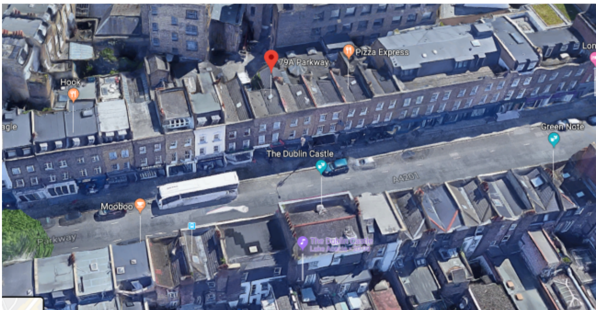
2) Birds eye view highlighting that the majority of roofslopes have been altered within the terrace
