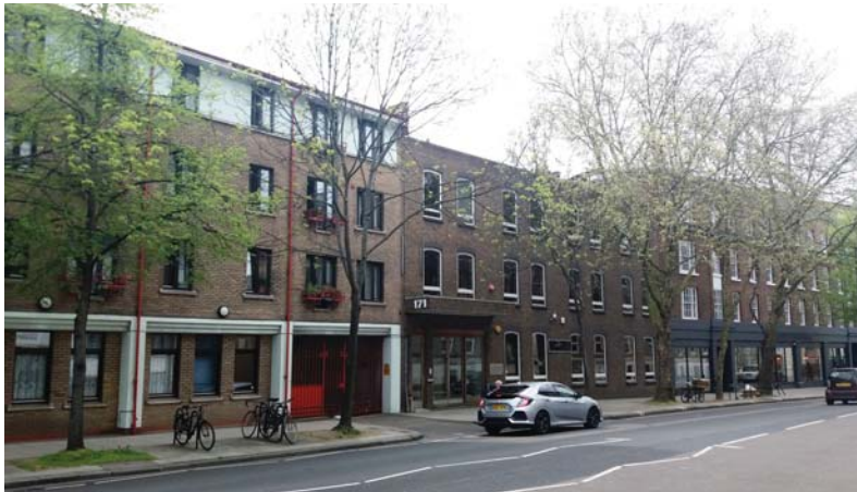
Front Street View from Gray's Inn Road looking North
