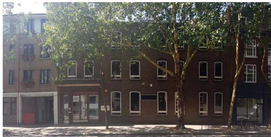
171-173 Gray's Inn Road Front Facade
