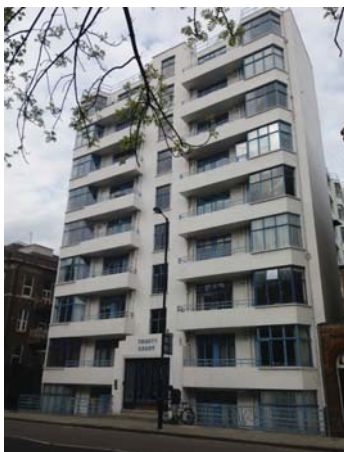
Trinity Court opposite from Site
