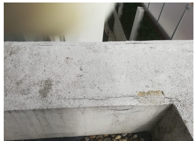
Detail showing delamination & water penetration of existing render
