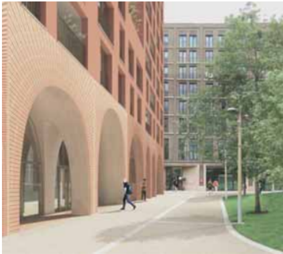
Figure 84: View showing the main entrance and lobby on Cubitt Park
