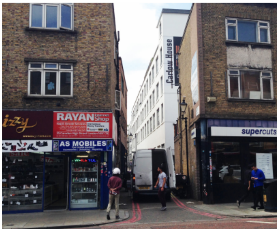
Photo 2: View of Symes Mews from Camden High Street
