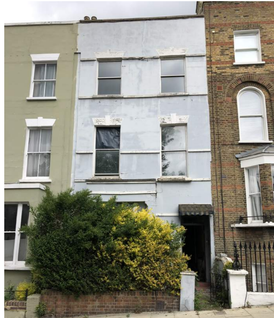
Front facade of the application site at street level.
