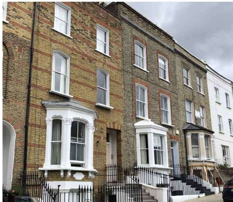
View of the Georgian properties west of the application site on Churchill Road
