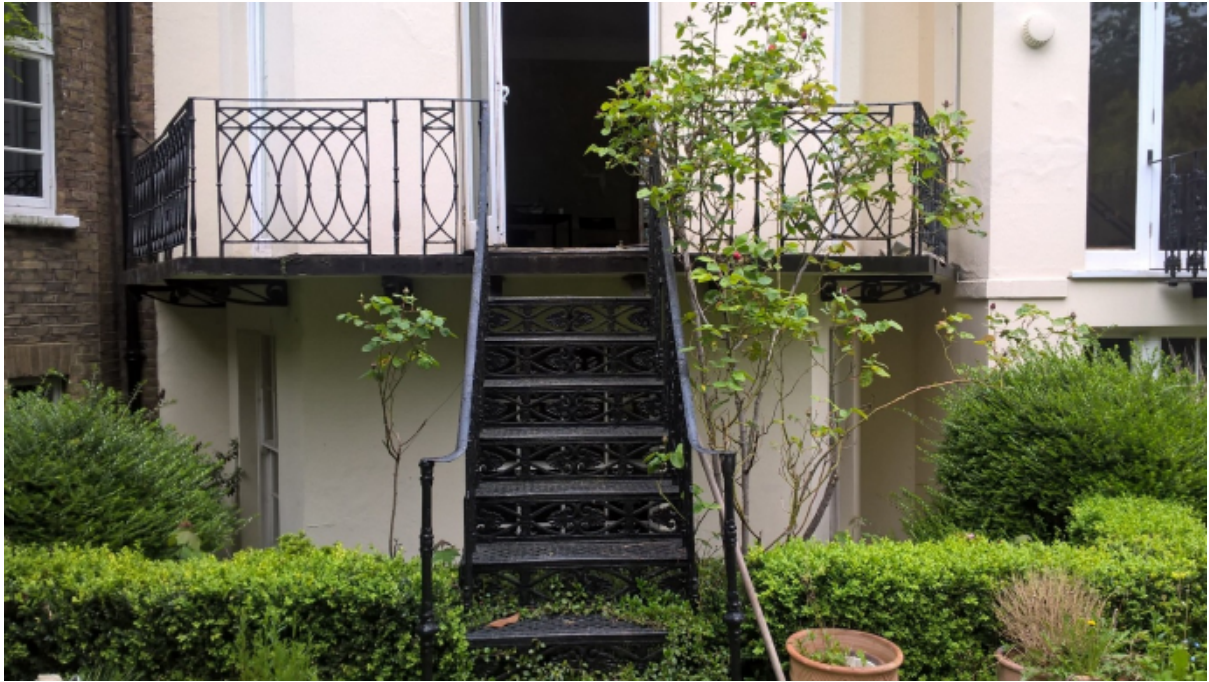
2. Cast iron steps to be widened and railings refurbished.
