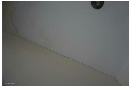
Rear Hall - Ceiling junction separation to the front
