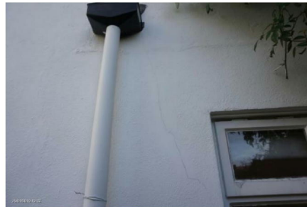
Right Elevation of Extension - Vertical crack
