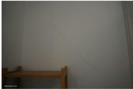
Bathroom - Diagonal crack to front wall
