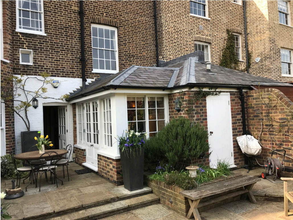
Photo of existing rear extension
