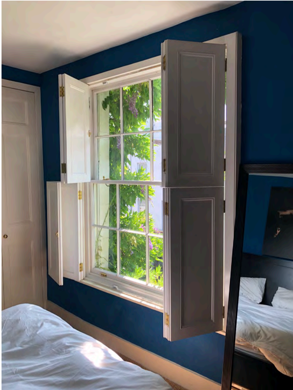
Figure 6: Internal view of window at second floor, to the east
