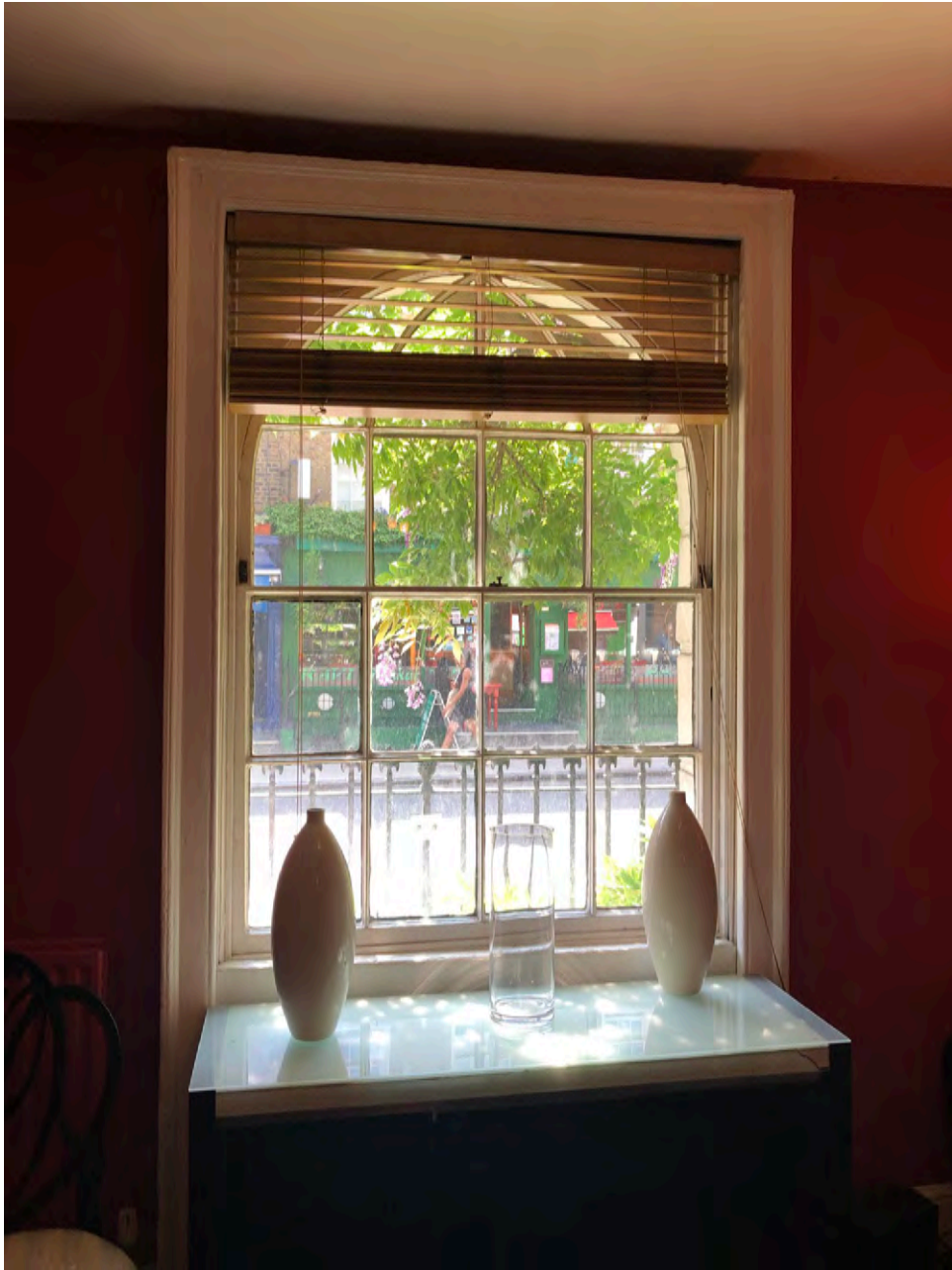
Figure 2: Internal view of window at ground floor level
