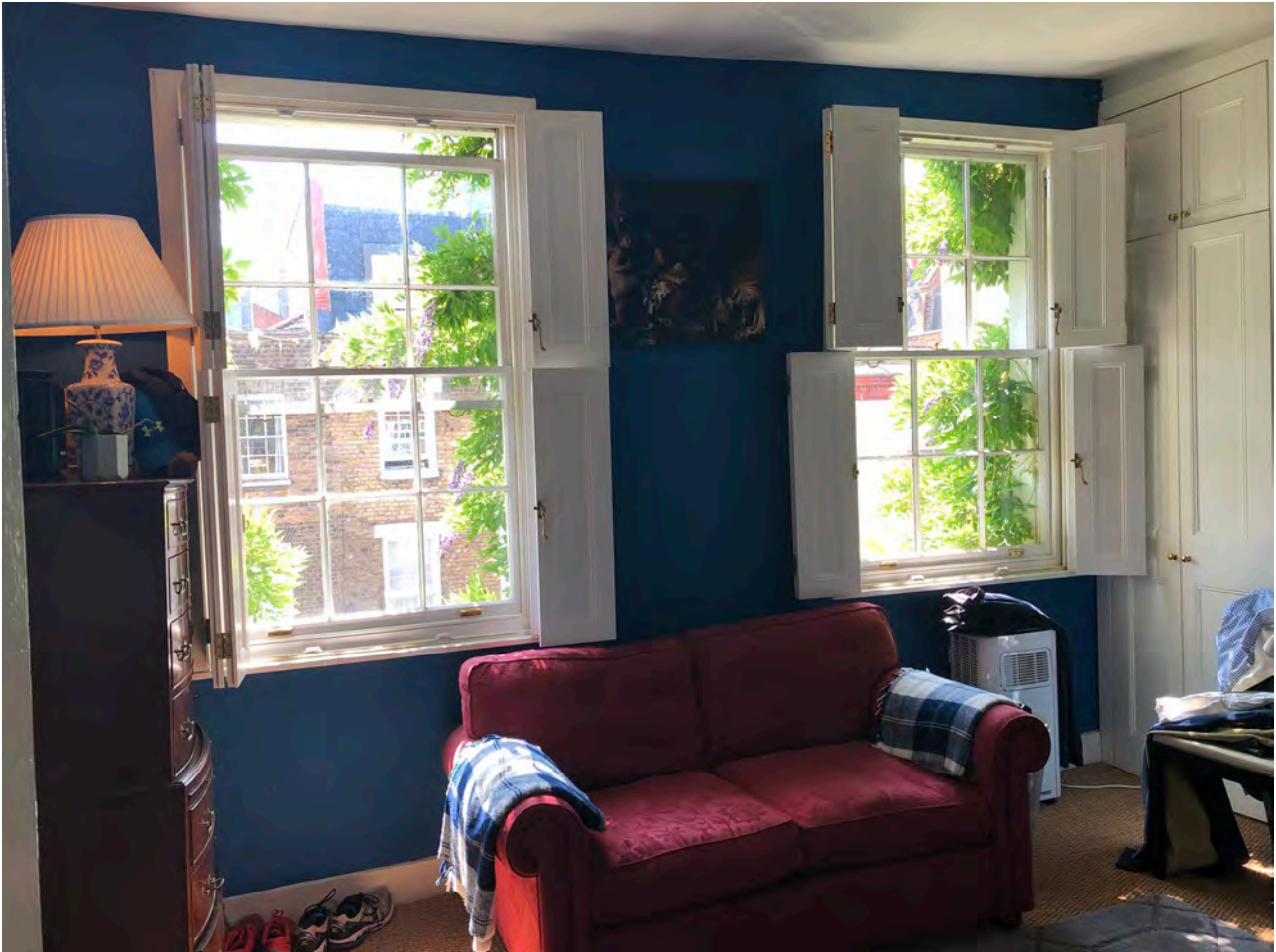
Figure 5: Internal view of windows at second floor, to the west
