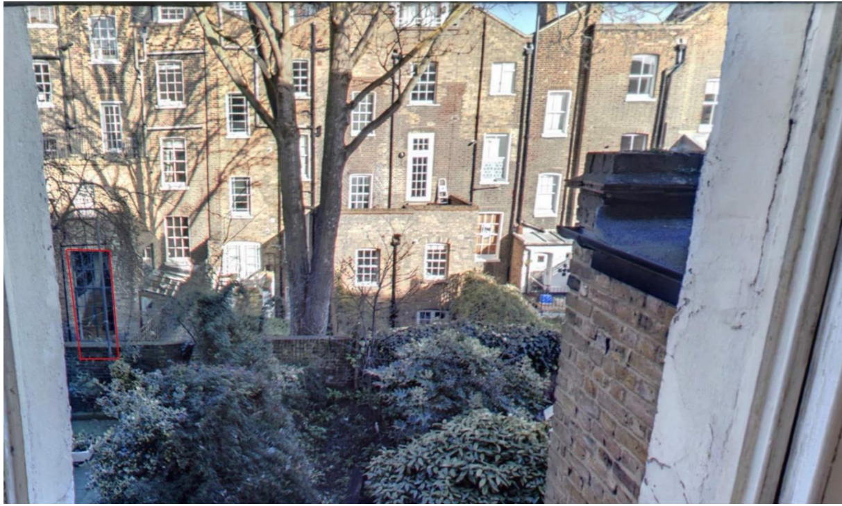
15 Albert Street double height window/door and excavated rear garden in a much smaller total garden area than No8 Mornington terrace
