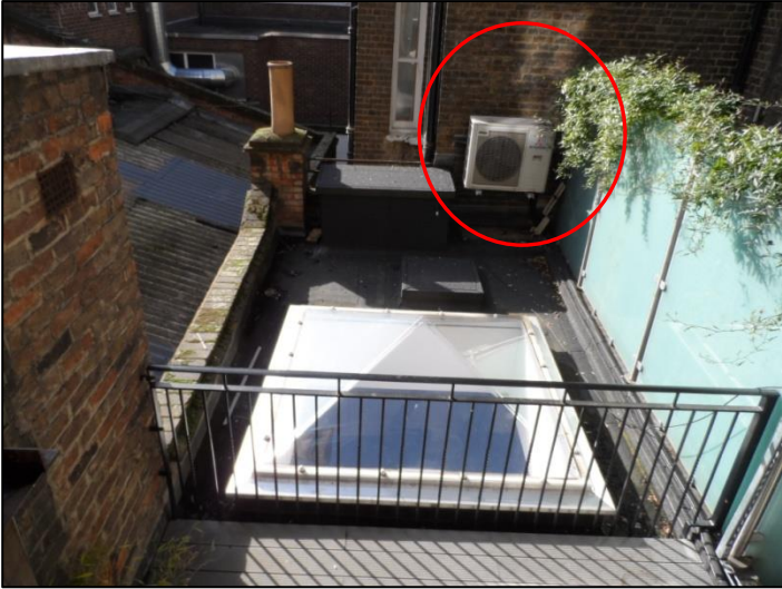
Figure 2 – Existing air condensing unit to be replaced – circled red.
