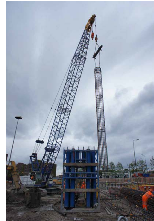
Figure 5.3 Installation of pile cage reinforcement (One Nine Elms, London)
