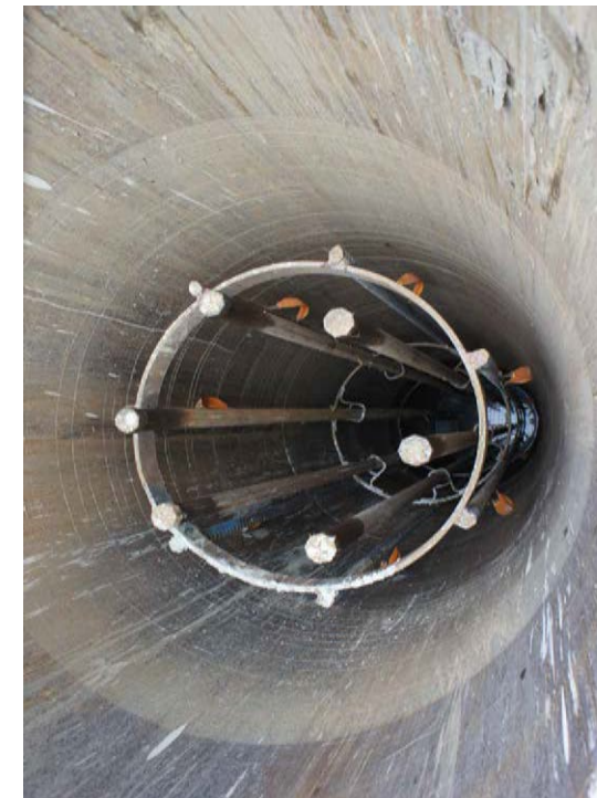
Figure 5.4 Pile cage reinforcement (One Nine Elms, London)
