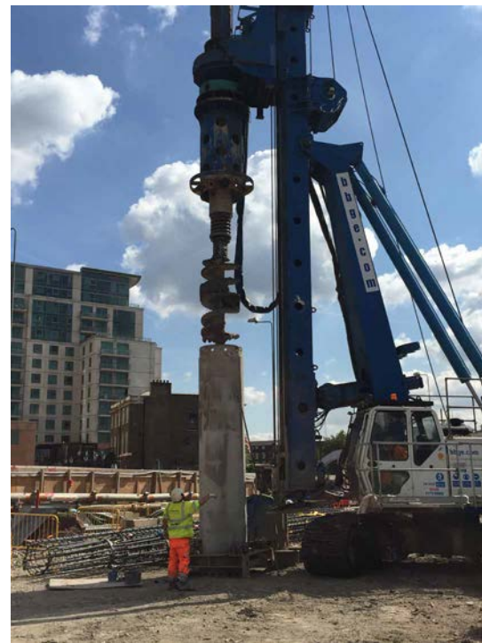
Figure 5.2 Steel encased rotary boring (One Nine Elms, London)
