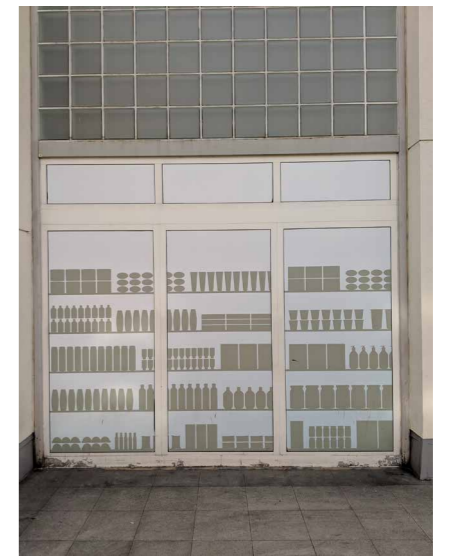
Current signage in-situ/Proposed signage location
