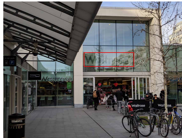
Current signage in-situ/Proposed signage location
