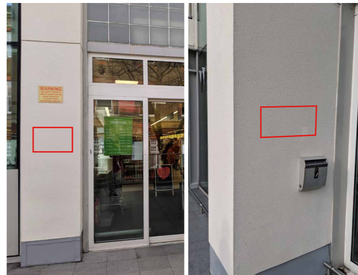
Current signage in-situ/Proposed signage location
