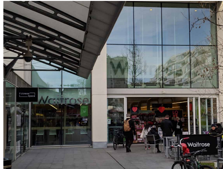
Current signage in-situ/Proposed signage location
