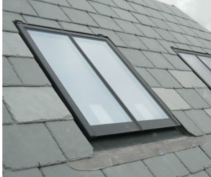
IMAGE PRECEDENT OF CONSERVATION ROOFLIGHT WITH TRADITIONAL VERTICAL GLAZING BARS IN BLACK METAL (FLUSH WITH ROOF SLATES)
