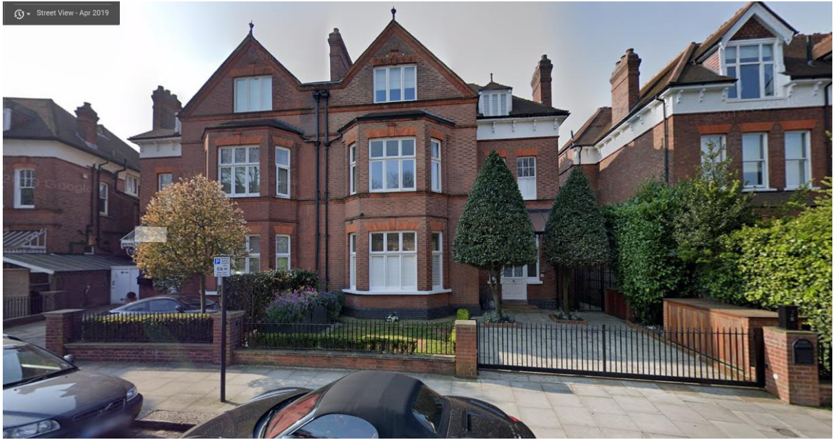
5. Street view of railings at Nos. 21-23
