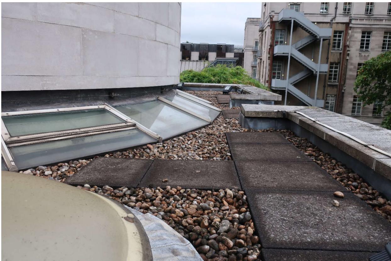
Figure 7-4 - Facing South-West over parapet from roof level
