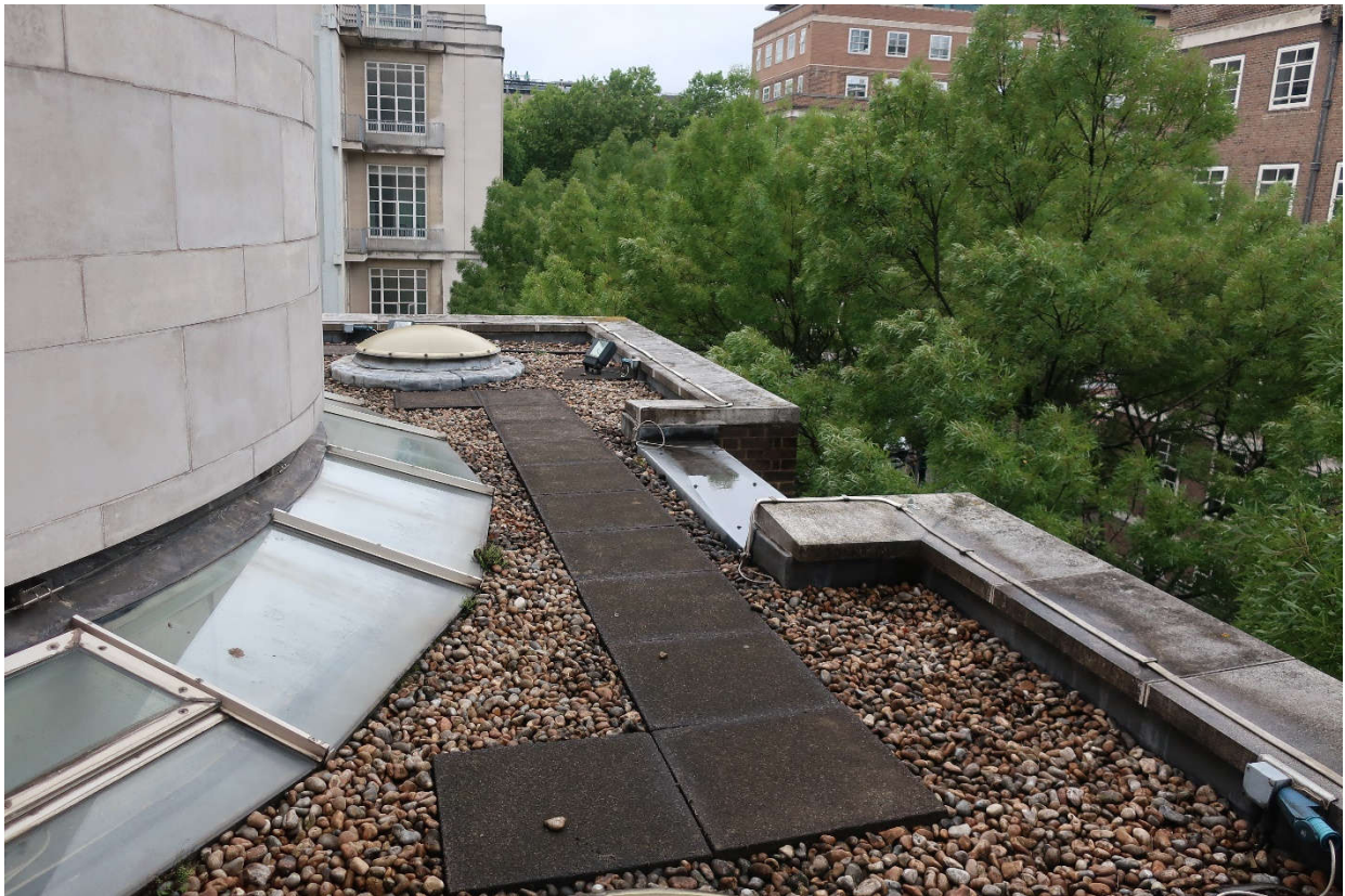
Figure 7-3 - Facing North-West over parapet from roof level
