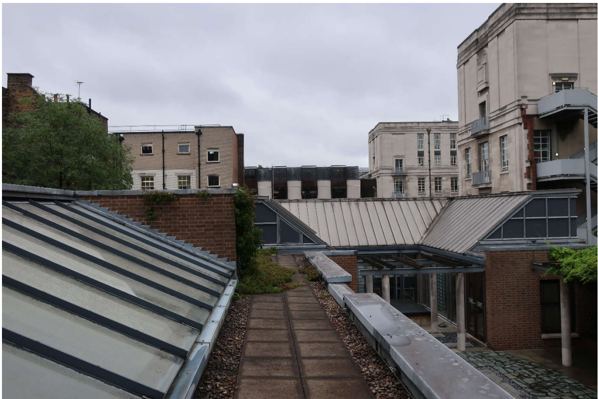
Figure 7-6 - Facing South on roof adjacent Japanese roof garden
