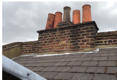
6. Existing butterfly roof and chimney stacks in relation to party wall between 269 and 271 Camden High Street
