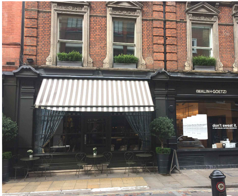
VIEW OF EXISTING No.8 MONMOUTH ST
