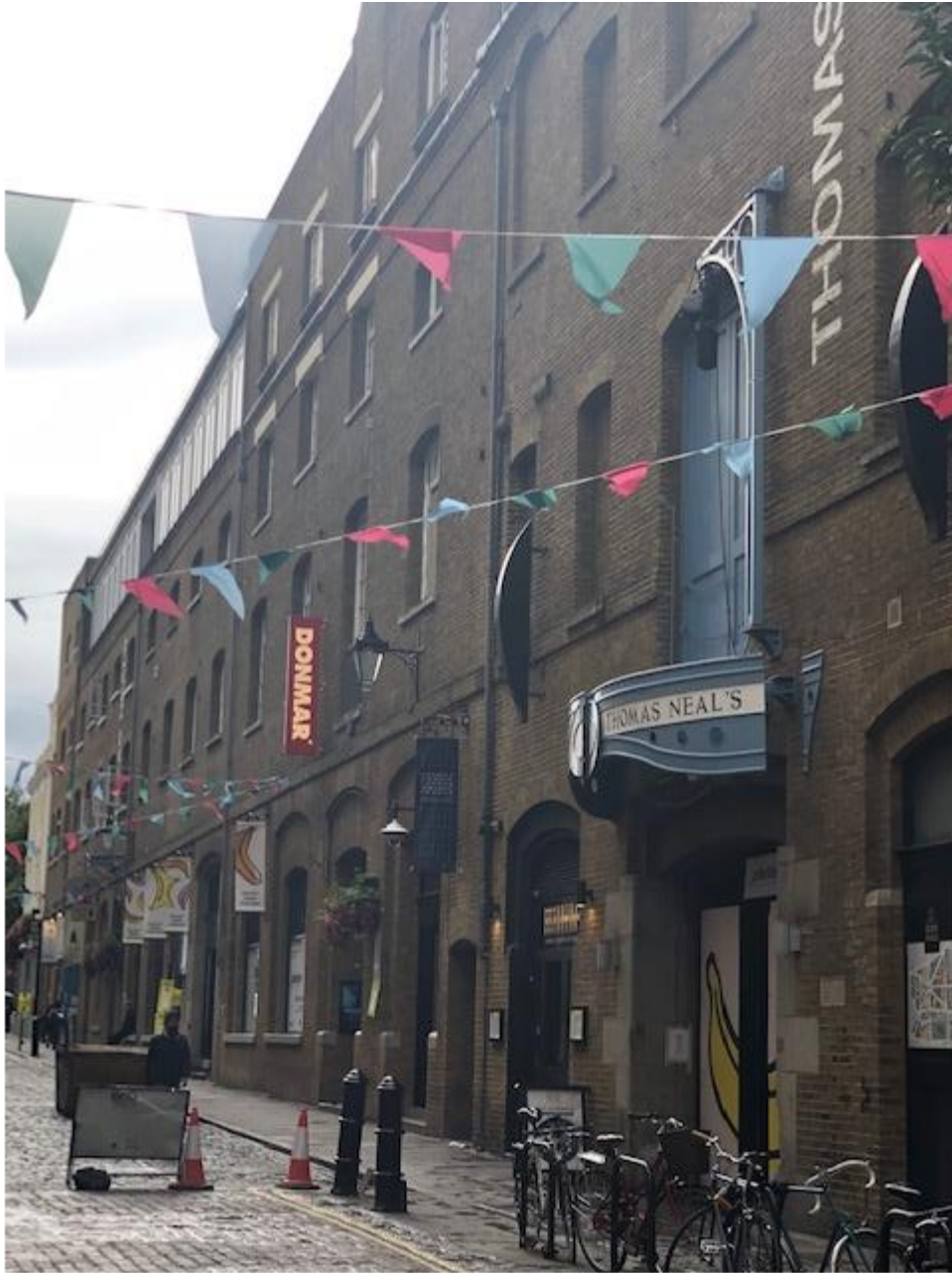
2. Earlham Street elevation with existing adverts.
