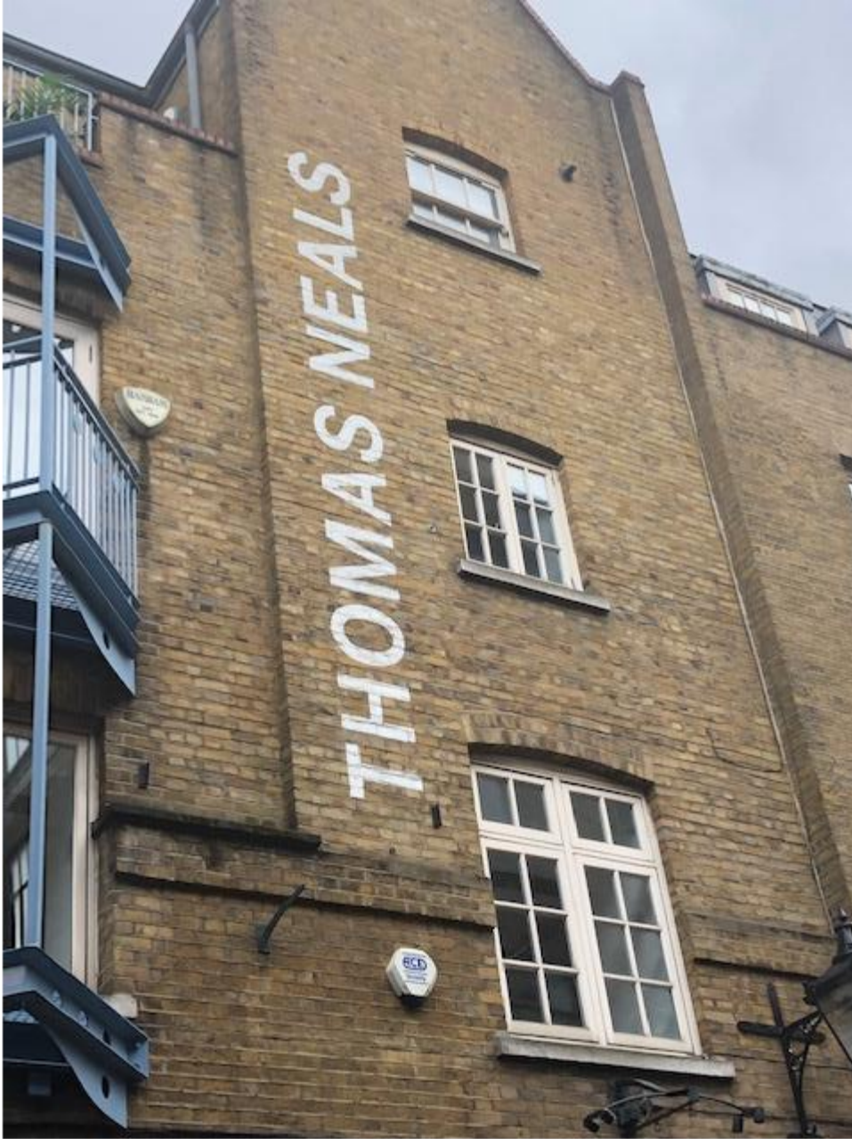
5. Existing painted signage.
