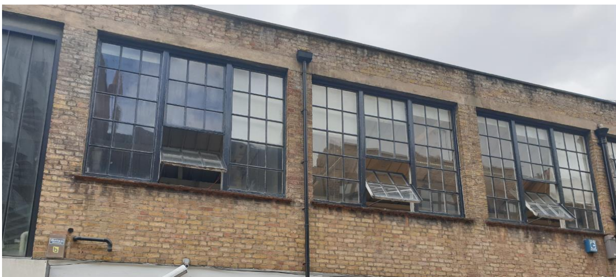
Figure 4 First Floor Brownlow Mews façade industrial Style Opening Windows
